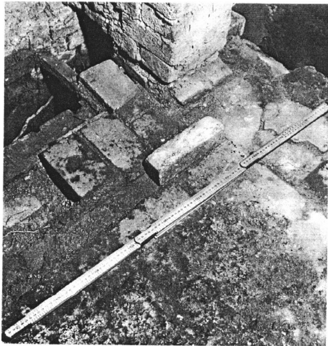
Fig. 8 The bed of the annealing furnace showing the groove from which sprang the muffle arch, and part of the firebox, top left. Scale, metre.
