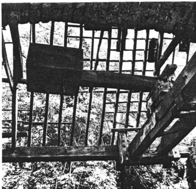
Fig. 14 The balance beam of the second partly ruined Saltford annealing furnace. This has now collapsed.
