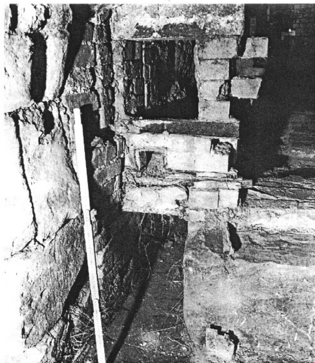
Fig. 11 Rear of annealing furnace showing door position and ashpit of left-hand firebox.
