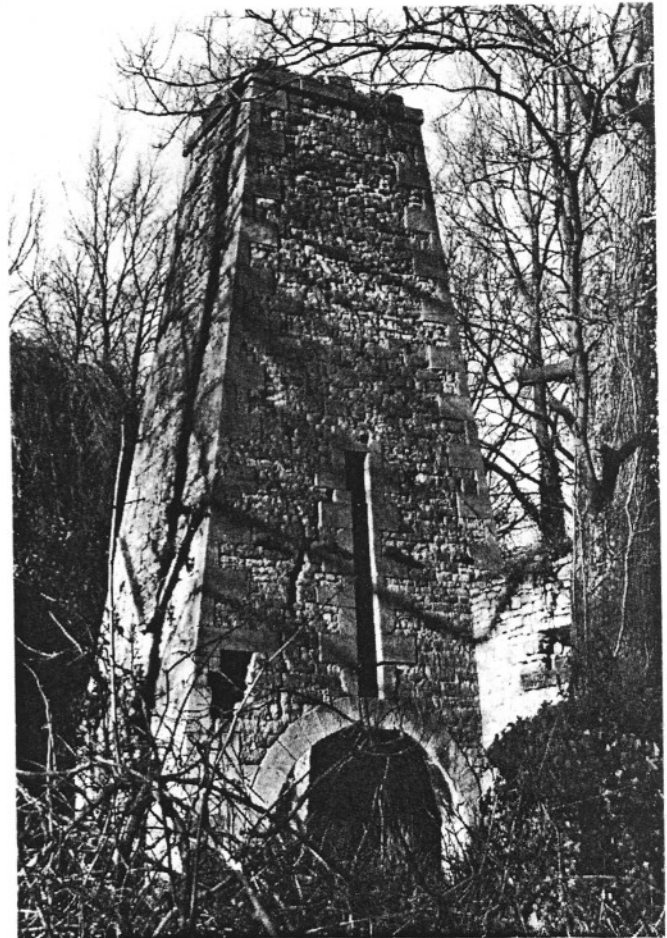
Fig. 13 One of the two shells of annealing furnaces surviving at Kelston. Of slightly different design to those at Saltford.
