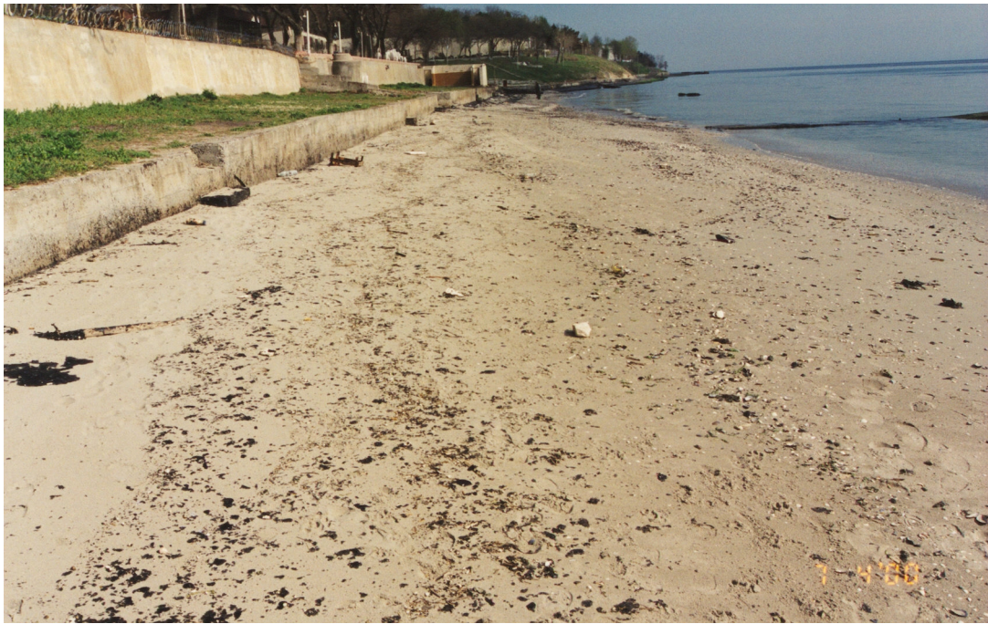
Figure 6b. Florya Municipality Recreation Facilities (7 April 2000)
