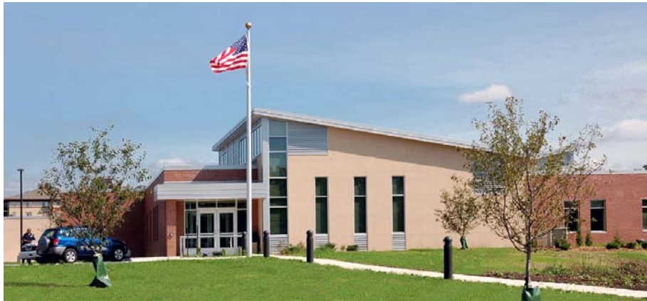
East District Station – Front View
