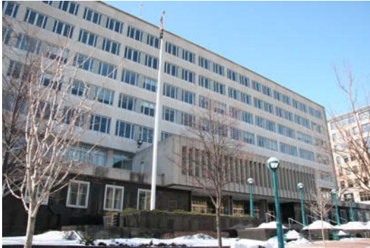
Central District Station/Administrative Offices
