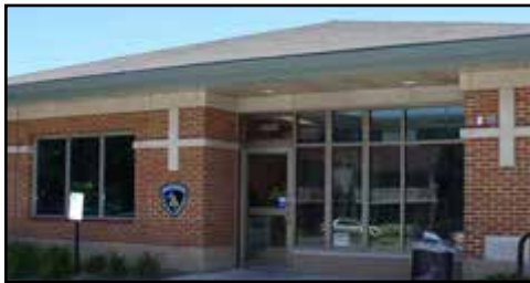
North District Station
