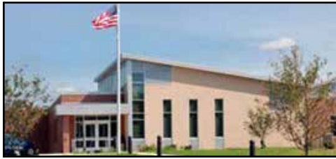
East District Station
