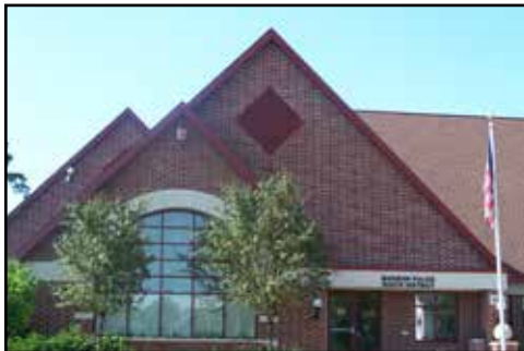
South District Station
