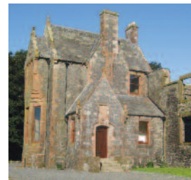
Restored porch at Glenlair in 2000
