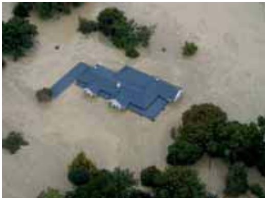
Many homes in rural areas of Manawatu Wanganui were overcome by floodwater in February 2004.
