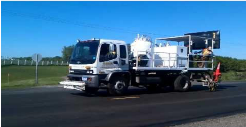
Figure L-1: Interim Broken Line Pavement Marking
