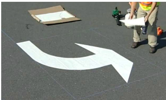
Figure H-2: Placement of Material
