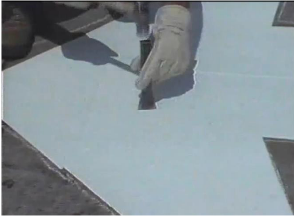
Figure H-4: Adhesion Test Being Performed
