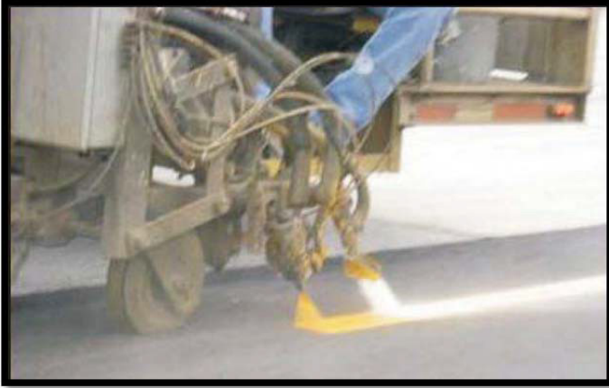
Figure E-8: Typical Bead Application
