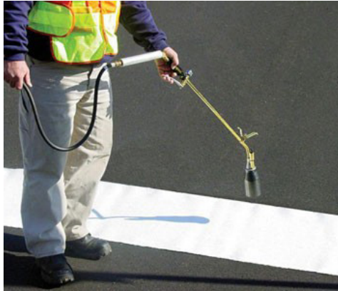
Figure H-3: Arrow Symbol Being Applied by Heat Torch
