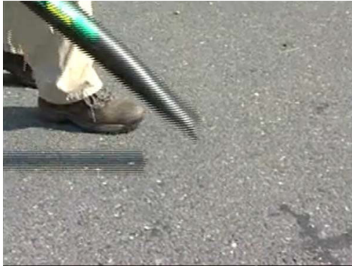
Figure H-1: Cleaning Pavement Prior to Application
