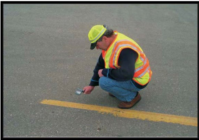
Figure O-3: Checking for Proper Bead Imbedment
