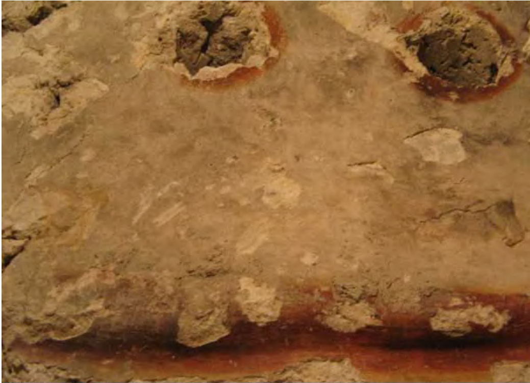
Figure 32b. Palace B-15: vault, soffit and holes for rafters.
