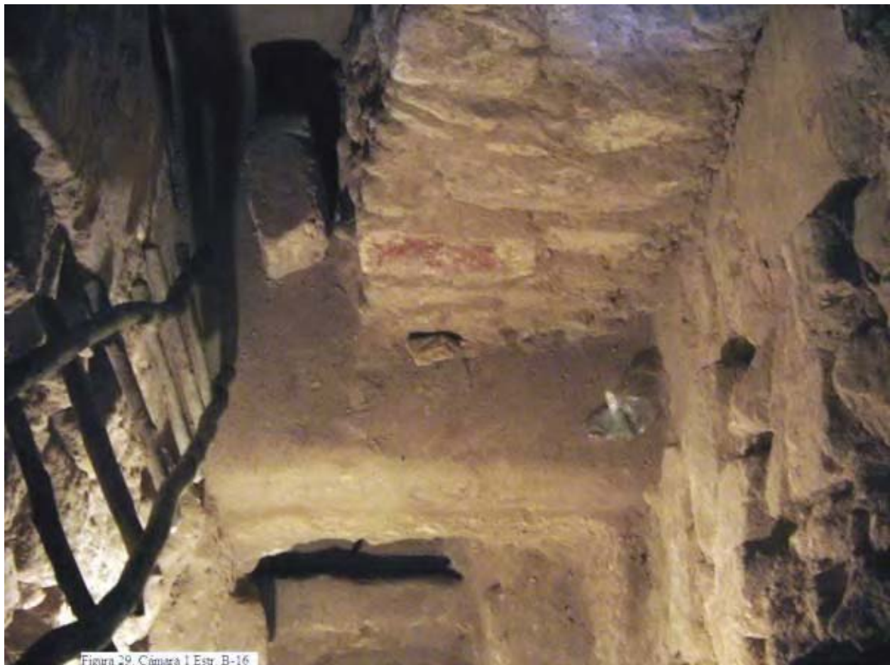
Figure 29. Chamber 1 of Structure B-16.
