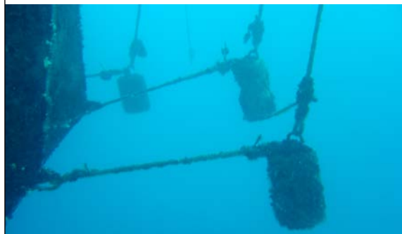
PLATE 32 Concrete sinkers installed incorrectly: the vertical sinker rope is too short and the net is hanging from the sinkers
