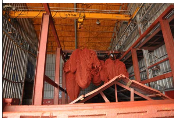
PLATE 77 A net treatment plant
