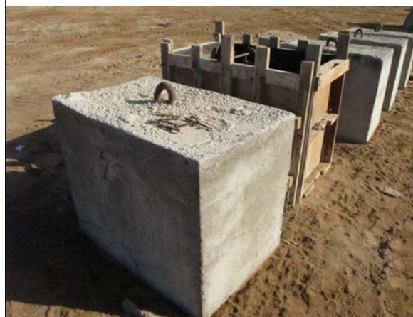
PLATE 7 Once the wooden form is filled with concrete, and the block has hardened, the form can be removed and the block left to dry for a few days
