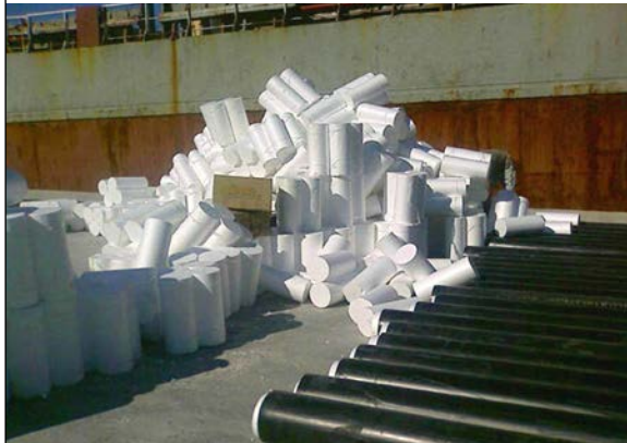
PLATE 40 Polystyrene cylinders are inserted into the pipes
