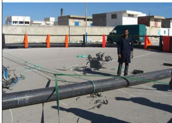
PLATE 42 Pipes are bent into a complete circle
