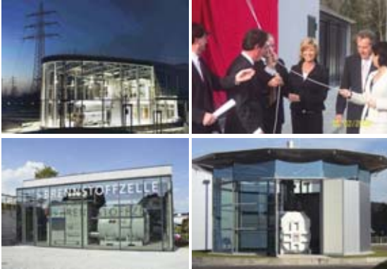
Folie 11 / MTU Onsite Energy
