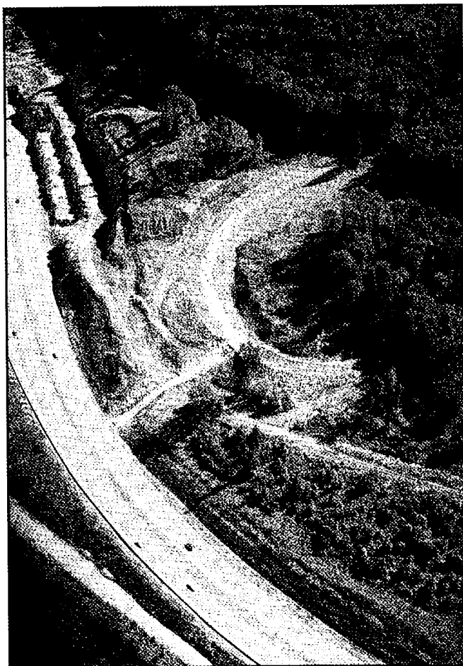
Figure 41. Debris deflection barrier (or berm) constructed to protect Trans-Canada Highway and Canadian National Railway rail track, 5 km southwest of Laidlaw in the Fraser Valley. GSC 1994-492E
