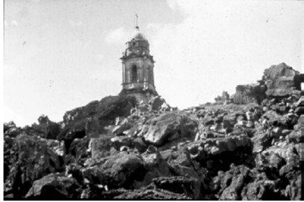
Blocky lava flow completely engulfs church at Paracutin, Mexico.
