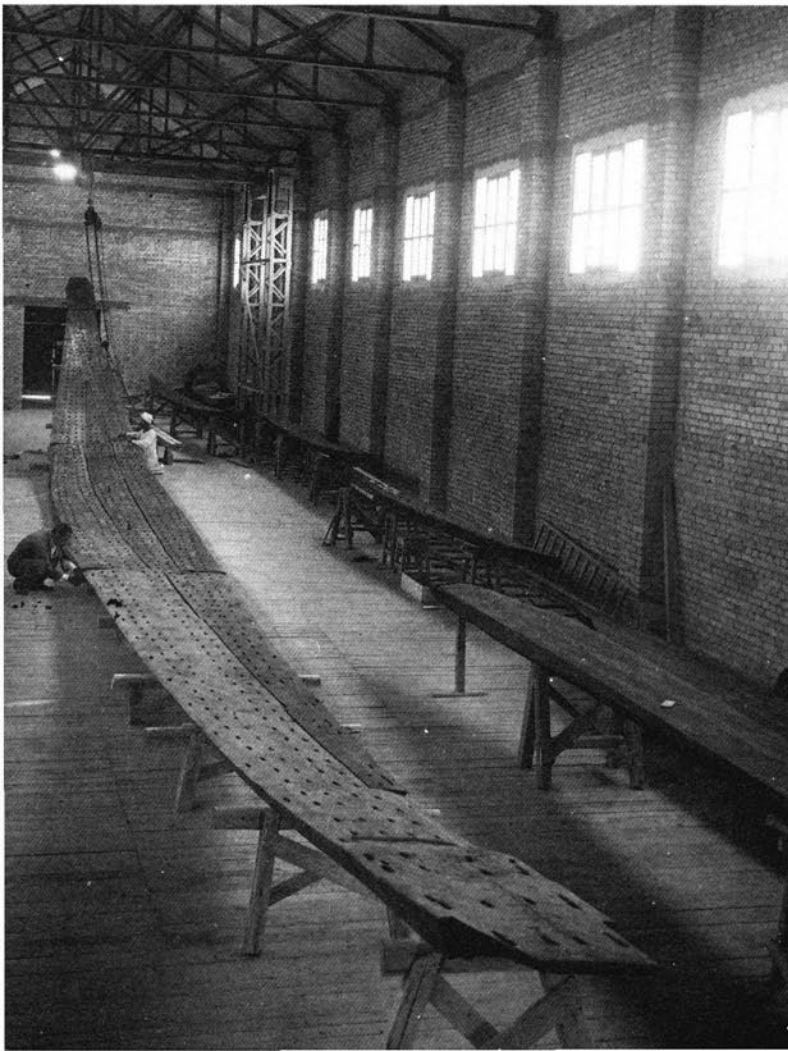
72 The bottom, or central, plank, was made up of eight timbers in three sections, forward, midships and aft. Laying out the timbers was fairly easy, but the difficulty came in determining how the three sections were related, particularly what their angles of abutment should be. On this depended the vital question of the bottom curvature, or fore-and-aft rocker, of the ship. Notice how much greater is the curvature at this stage than it was in ill. 61.
