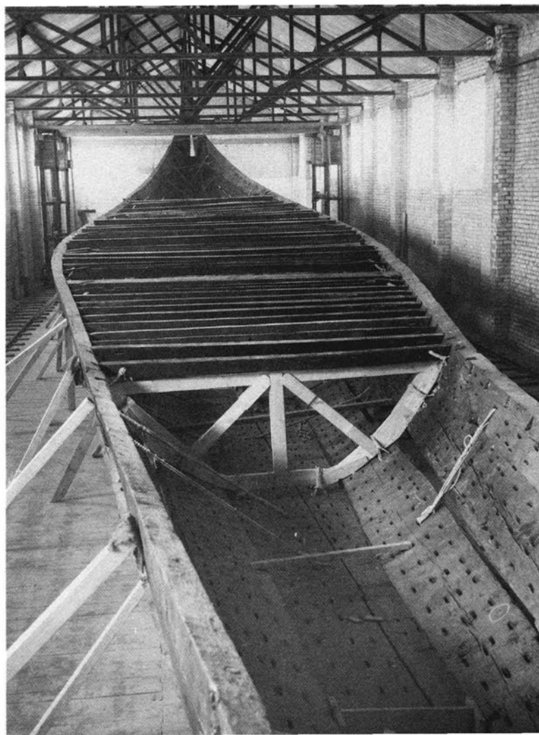
76, 77 Once the silhouette and section profile of the boat were understood it was possible to make template moulds around which the skin of hull timbers was erected. When the hull structure was complete, the moulds, having served their function, were removed.
