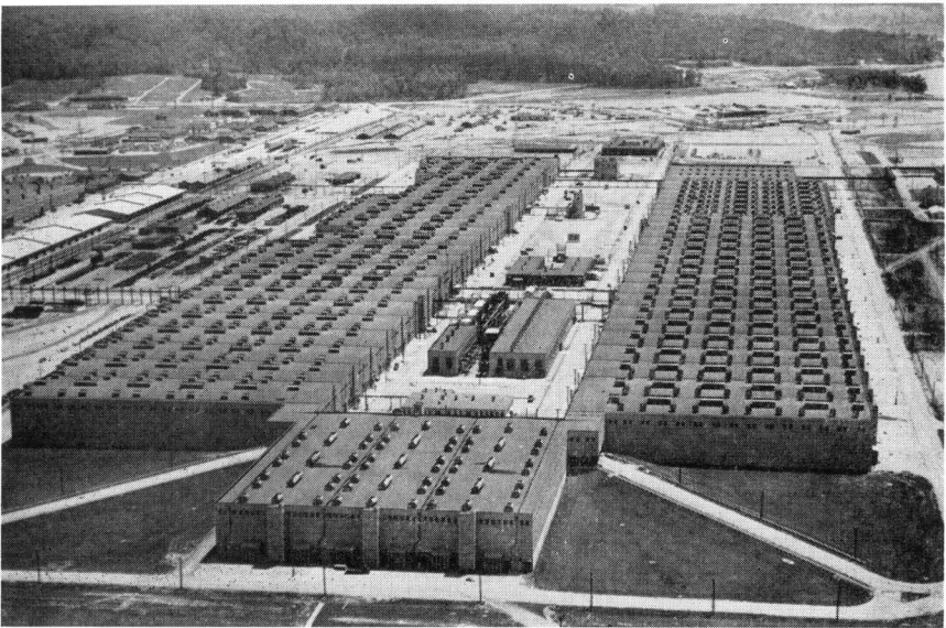
K-25, THE COMPLETED GASEOUS-DIFFUSION PLANT / This four-story structure was almost one-half mile long and almost 2 million square feet in area.
