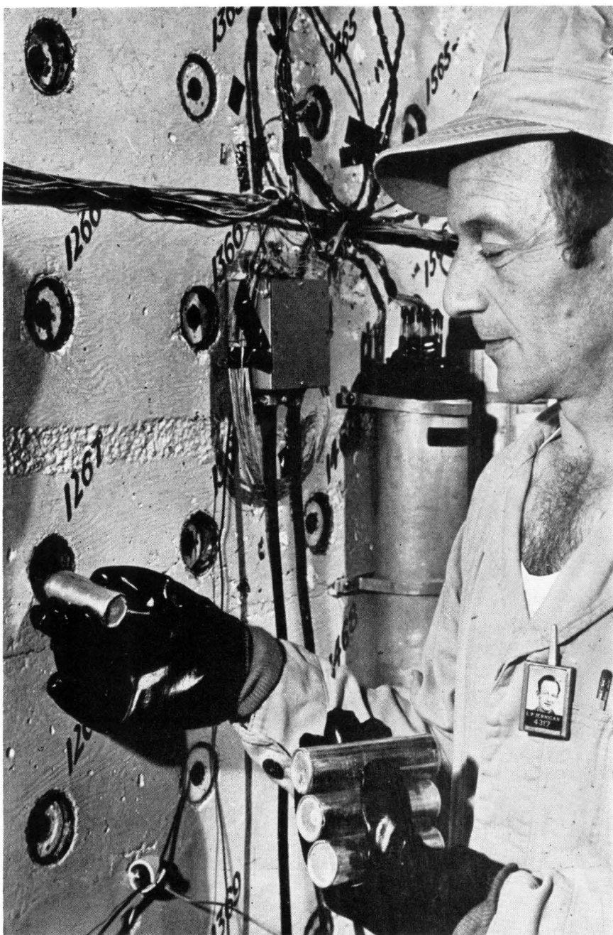
LOADING X-10 / The worker is inserting the aluminum-clad, natural-uranium slugs.
