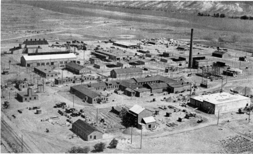
300 AREA AT HANFORD / Here du Pont manufactured uranium slugs and tested materials for the production piles. Slugs were fabricated in the one-story masonry building in the center background. Materials were tested in a 30-watt pile in the large vented building at the upper left.
