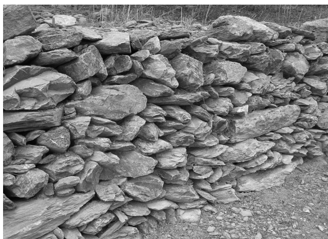
Fig. 6. Modern stone fence built of blue-green schist at the exit of Achlada towards Fodele.
