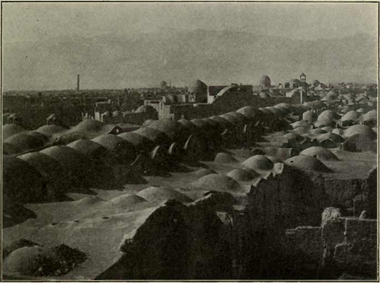
DOMED ROOFS OF KASHAN
