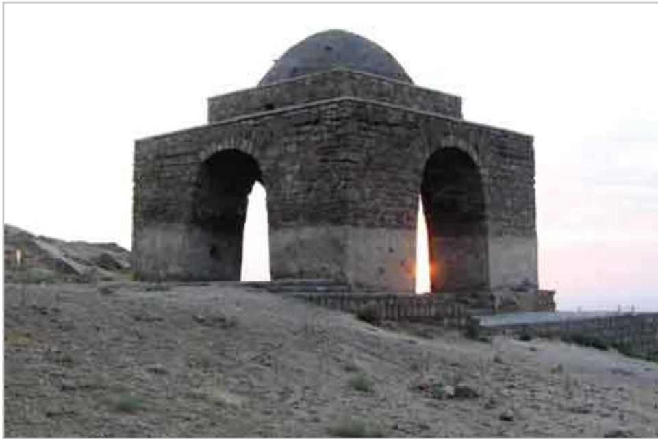
Sassanian chahar-taqi at Niasar near Kashan, Esfahan (Isfahan).
