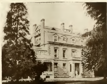
FRONT VIEW—MAIN BUILDING.
