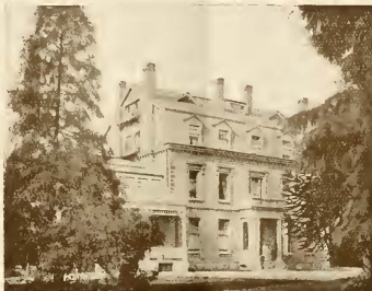
FRONT VIEW—MAIN BUILDING.
