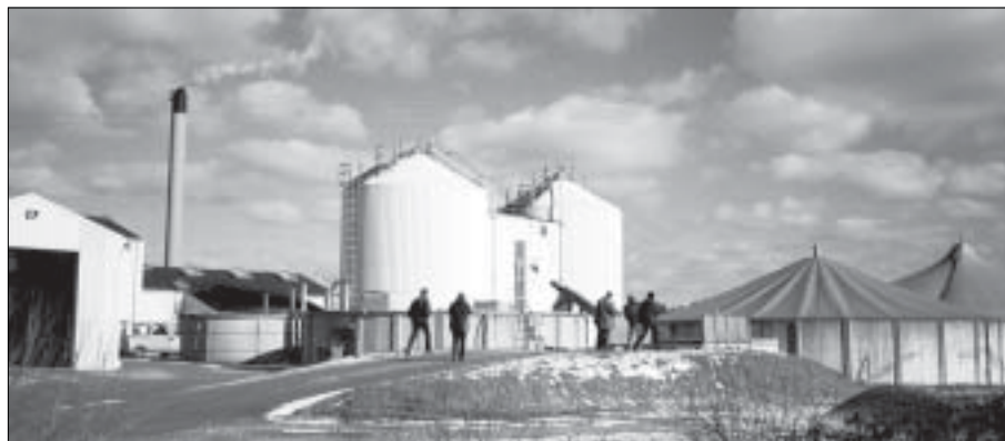
Visiting a biogas plant in Filskov during the study tour in Denmark. The plant receives slurry from 11 livestock farms, and the biogas is powering a 375-kW engine.
