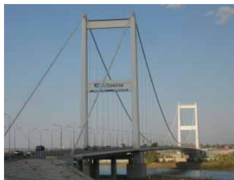
Irtys River Suspension Bridge
