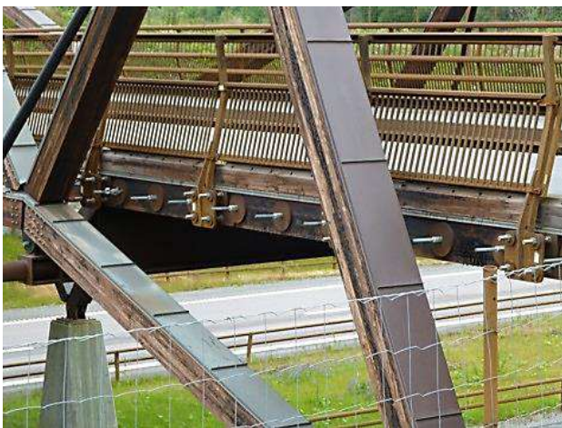
Figure 4-29: Sletta Bridge in Eidsvol, Norway. The structure consists of asymmetrical glulam trusses which carry steel crossbeams and a stress laminated deck. In addition to being dual preservative treated (with a copper-based preservative and creosote) the main elements are sheltered from moisture using metal flashing.
