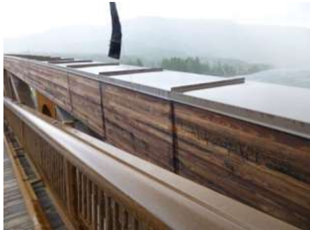
Figure 4-31: Tretten Bridge is a continuous truss across three spans. The truss is a hybrid truss made primarily from glulam timbers with steel vertical web members and steel shoes at the nodes. Corten weathering steel was used for the steel elements.
