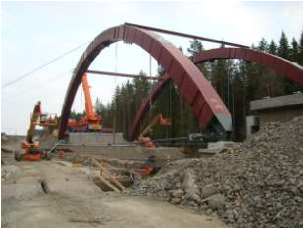
Figure 4-37: Nissan River Bridge spans 47.4m (155ft) and consists of two three-pinned arches. The arches carry steel hangers and crossbeams which in turn carry a stress-laminated deck. The glulam arches are sheltered by steel flashing on top and vented wood panels on the vertical faces.
