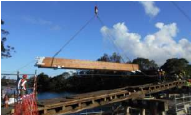
Figure 4-41: The new glulam superstructure and deck were installed on the existing substructure at Newry Island Bridge. Removal of the existing structure and installation of the new occurred in tandem to limit the road closure time.
