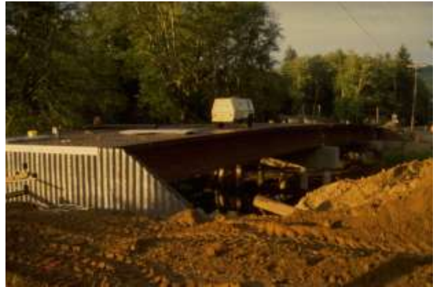
Figure 4-27: The Lighthouse Bridge, under construction in Clallam Bay, Washington. The bridge consists of six fiber-reinforced glulam girders in each span.
