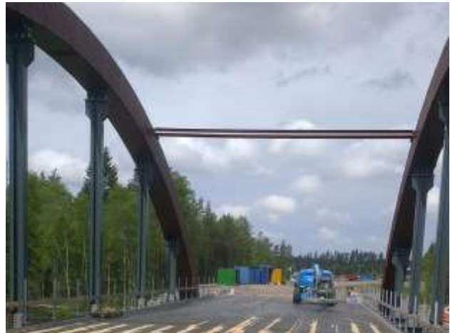
Figure 4-37: Nissan River Bridge spans 47.4m (155ft) and consists of two three-pinned arches. The arches carry steel hangers and crossbeams which in turn carry a stress-laminated deck. The glulam arches are sheltered by steel flashing on top and vented wood panels on the vertical faces.
