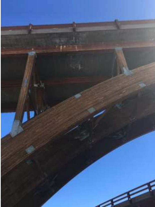
Figure 4-3: The upper bridge is supported by glulam arches.
