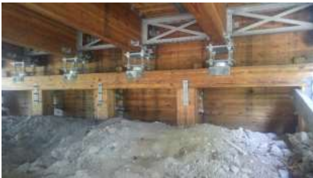
Figure 4-21: Snake Road Bridge, on the border between Hamilton and Burlington, Ontario, consists of six glulam girder lines. The substructure was completely rebuilt; however, much of the material from the original structure was salvaged for use in the new bridge. The substructure was completely timber and the highway was designed for two lane heavy truck use beyond a conventional CL625 rating. It also incorporated an all timber TL4 truck crash proof rail system.
