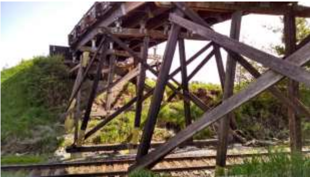
Figure 4-20: Providence Road Bridge in Clarington, Ontario consists of five lines of glulam girders supporting a transverse timber deck. The existing solid sawn frame bents were restored, including the addition of high-strength fiber reinforcing in some locations to restore capacity that had been lost due to decay. An asphalt wear surface was installed on top of the transverse timber deck. The timber guard rail is crash-tested to TL-4 specifications.
