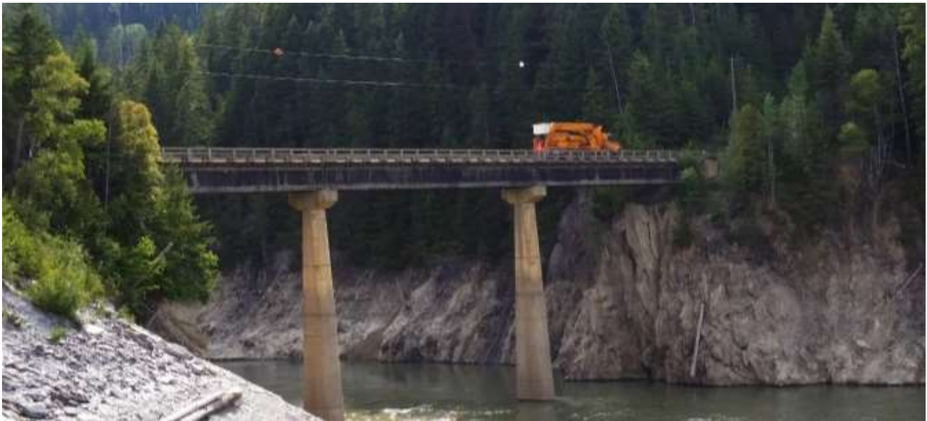
Figure 4-5: Golden Bridge, in British Columbia is a 3-span glulam timber bridge, totaling 82m (270 ft) in length.
