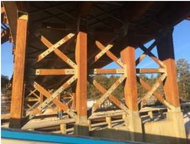
Figure 4-4: The substructure of the lower bridge consists of glulam timber frame bents.
