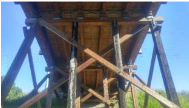
Figure 4-22: Dickinson Road Bridge, in Port Hope, Ontario consists of six glulam girder lines. The substructure was completely rebuilt; however, much of the material from the original structure was salvaged for use in the new bridge.
