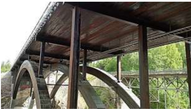
Figure 4-34: Asta Bridge is a stress laminated deck supported by glulam arches. The deck totals 96.6m (317ft), and the arches span 38.5m (126ft).
