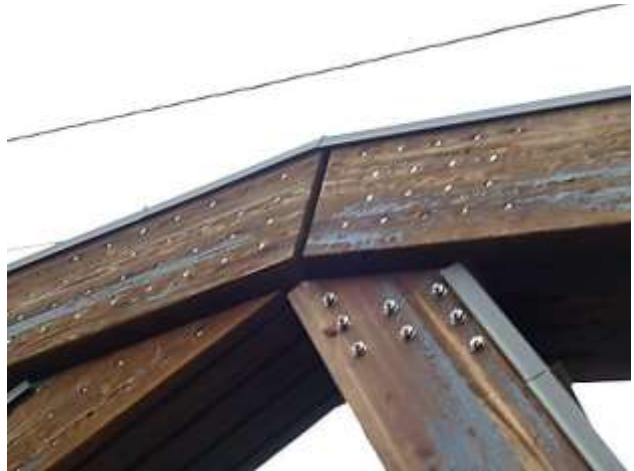
Figure 4-29: Sletta Bridge in Eidsvol, Norway. The structure consists of asymmetrical glulam trusses which carry steel crossbeams and a stress laminated deck. In addition to being dual preservative treated (with a copper-based preservative and creosote) the main elements are sheltered from moisture using metal flashing.
