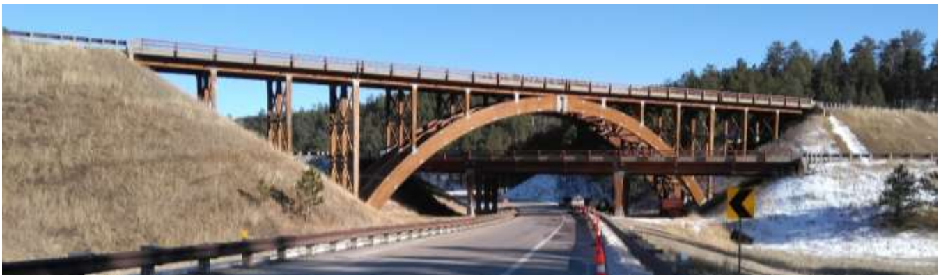
Figure 4-2: The wye includes an upper bridge supported on three-pinned glulam arches, and a lower three-span bridge supported by glulam girders.
