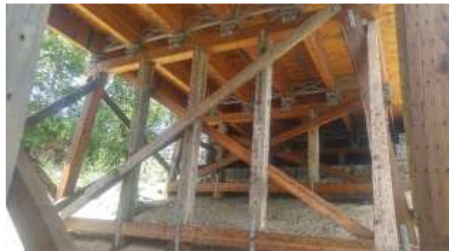
Figure 4-21: Snake Road Bridge, on the border between Hamilton and Burlington, Ontario, consists of six glulam girder lines. The substructure was completely rebuilt; however, much of the material from the original structure was salvaged for use in the new bridge. The substructure was completely timber and the highway was designed for two lane heavy truck use beyond a conventional CL625 rating. It also incorporated an all timber TL4 truck crash proof rail system.
