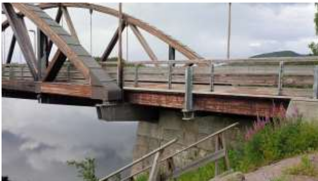
Figure 4-35: Flisa Bridge is a three-span glulam truss bridge totaling 196m (643ft) with a maximum span of 70m (230ft).
