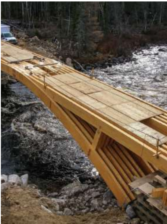
Figure 4-26: Tamiscame River Bridge, by Nordic Structures, consists of 12 glulam arches spanning 30m (98ft) which support 10 glulam girders and a transvers glulam deck. (Forestrie Nordic, 2015)
