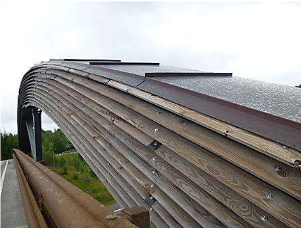
Figure 4-30: Skogsrud Bridge in Tangen, Norway consists of two glulam arches and a stress-laminated deck. The arches are protected with metal flashing on top and wood louvers on the vertical faces. This shelters the elements from rain while still allowing sufficient air flow to keep the moisture content of the wood low.
