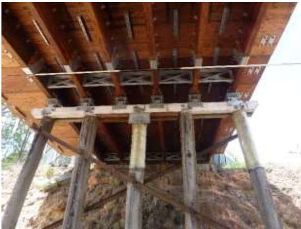
Figure 4-40: Boundary Road Bridge is a four-span overpass crossing a pair of Queensland Rail tracks. The light weight of the timber superstructure allowed each span to be preassembled alongside the road and lifted into place by crane. This limited the interruptions to rail traffic on the tracks below. This bridge was installed in 41 hours.
