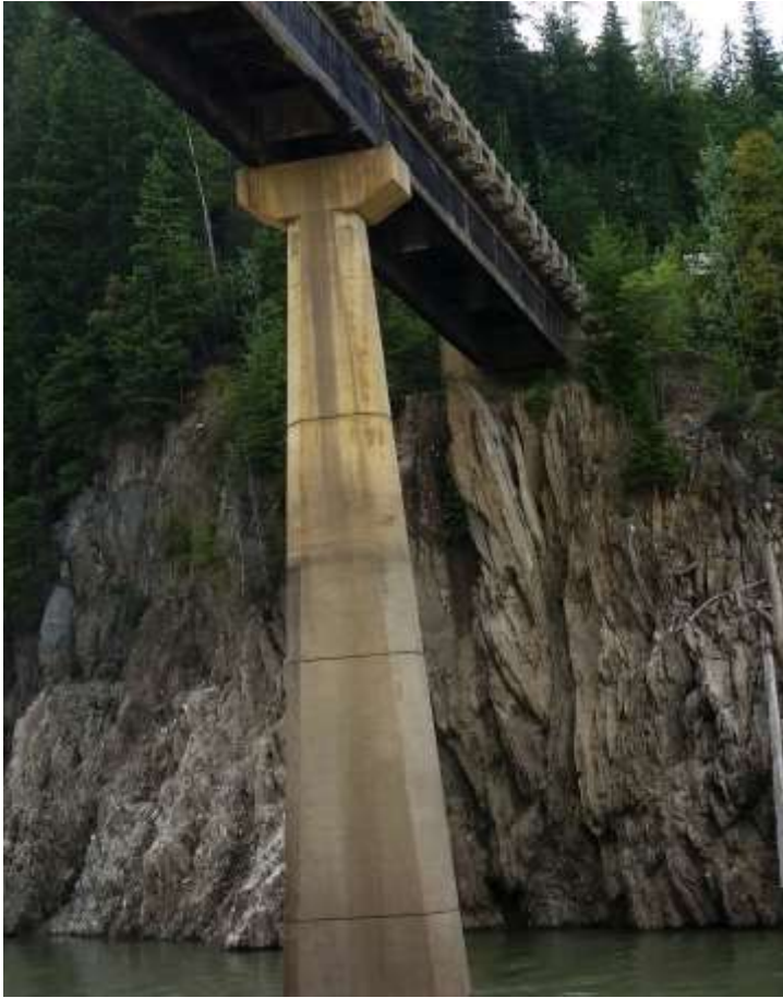
Figure 4-6: Each 27m (90 ft) span consists of two glulam I-Beams which support transverse bearers. The deck and wear surface are made up of longitudinal planks.
