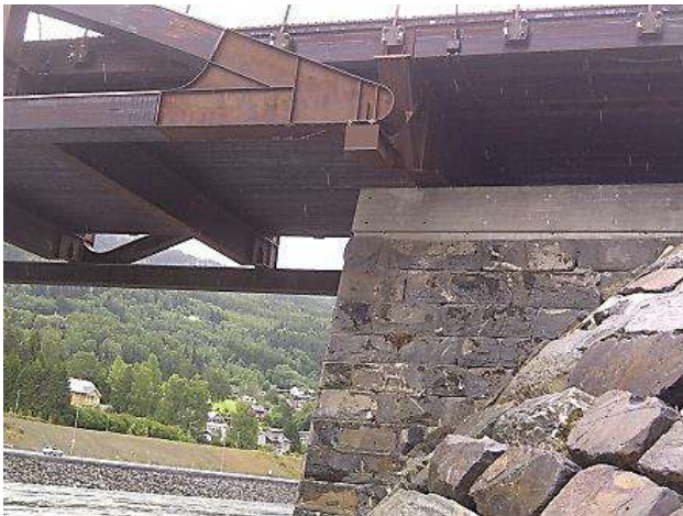
Figure 4-31: Tretten Bridge is a continuous truss across three spans. The truss is a hybrid truss made primarily from glulam timbers with steel vertical web members and steel shoes at the nodes. Corten weathering steel was used for the steel elements.
