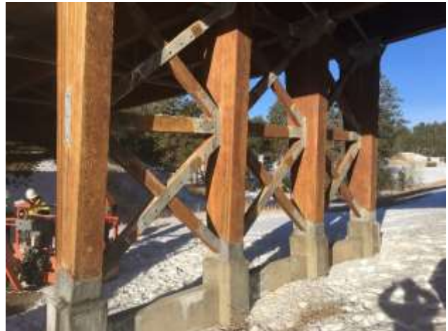
Figure 4-4: The substructure of the lower bridge consists of glulam timber frame bents.
