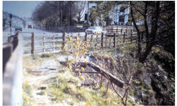
Figure 31: Tram tracks in the air in 1984.
