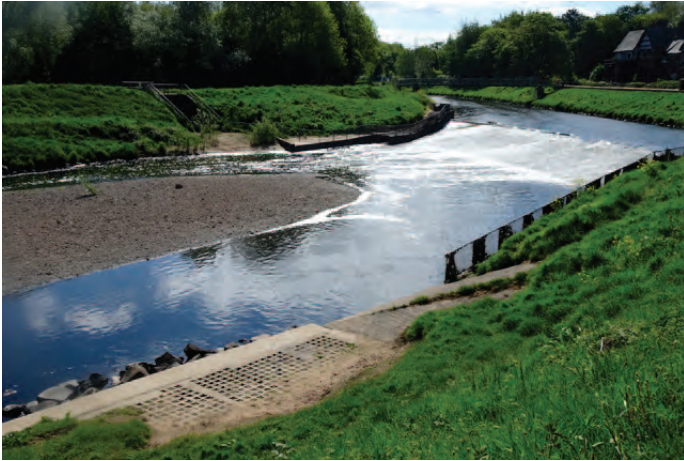
Figure 7: The embankments, weir and gravel bar on the Mersey at Mill Lane, Northenden in 2020.
