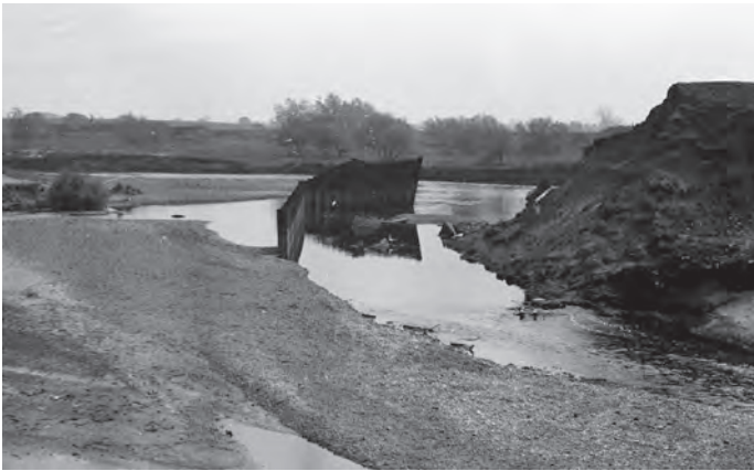
Figure 11: The Mersey at Urmston in March 1983 (left) and Figure 12: in early 1986 (right) showing how shift to the channel caused the iron piling installed to protect the pylon on one bank ended up on the other side of the channel.
