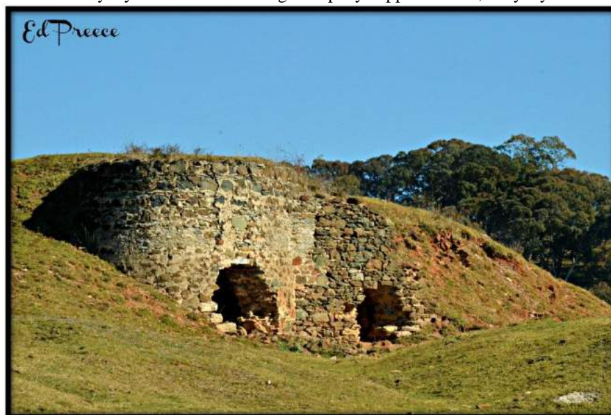
Figure 1. Remains of the Blayney Mines and Smelting Company copper smelter, Blayney NSW.
