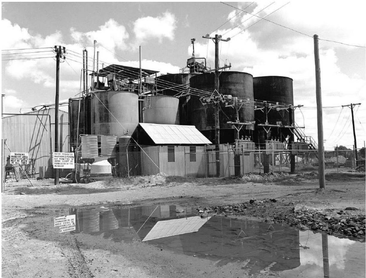
Figure 15: The first cyanide CIP plant built in Australia, at Mount Boppy, by Leighton Mining NL in 1974. Source: NSW Geological Survey Photo Collection, photograph taken by G. Hicks.
