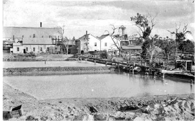
Figure 21: Treatment plant and slime pits Mount Boppy mine, 1905.
