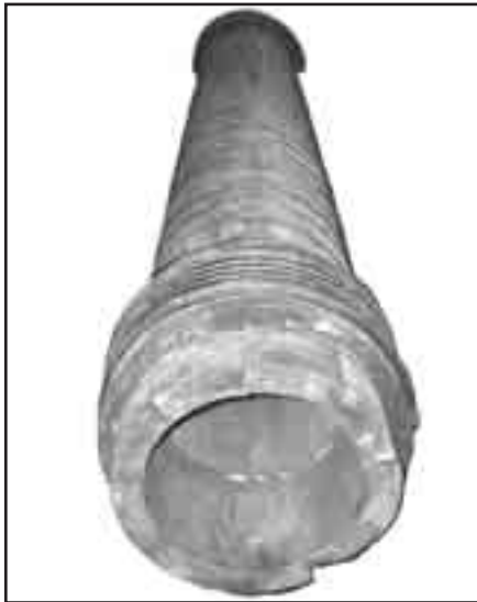
▲ Wooden Water Main
