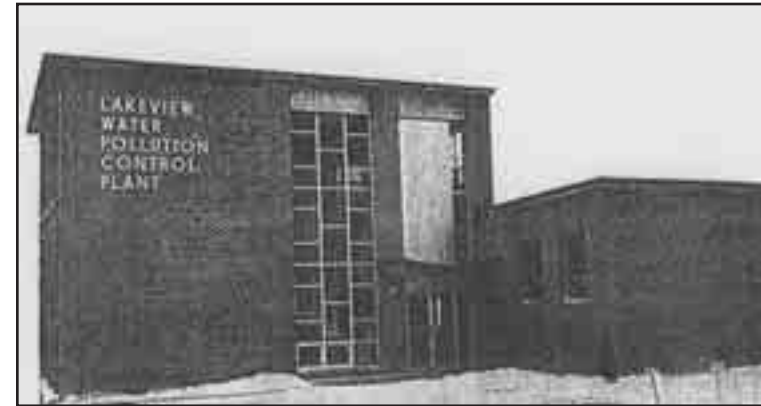
▲ Lakeview Water Treatment Plant
