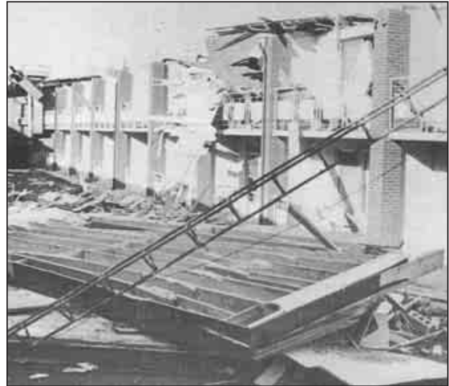
▲ Damaged Aero Inn
