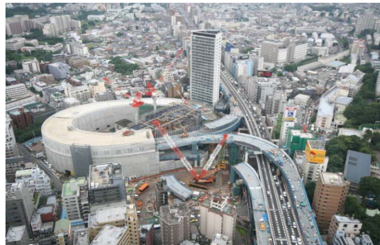
Construction of viaduct in an urban setting
