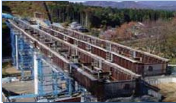
Bridgework in a mountainous area
