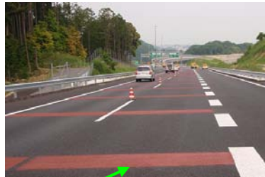
Rough layer of pavement
