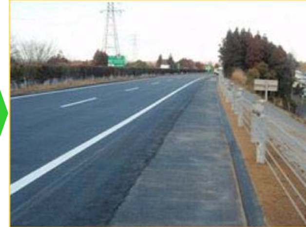
Re-open to traffic (6days after the quake)
