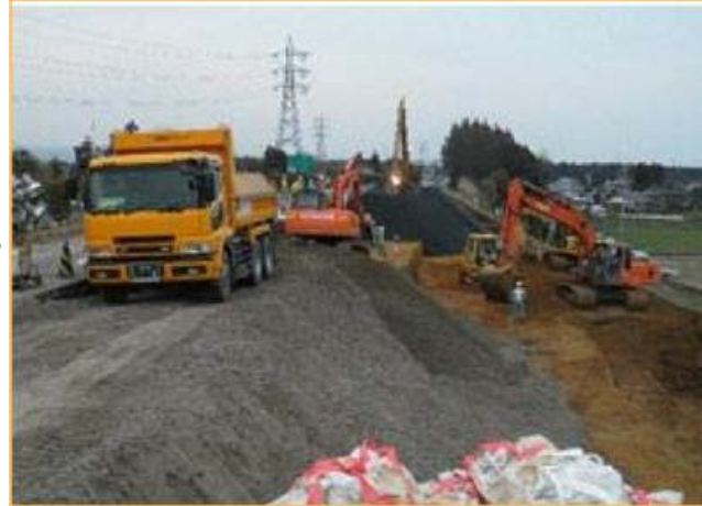
Restoration work 3 days after the earthquake
