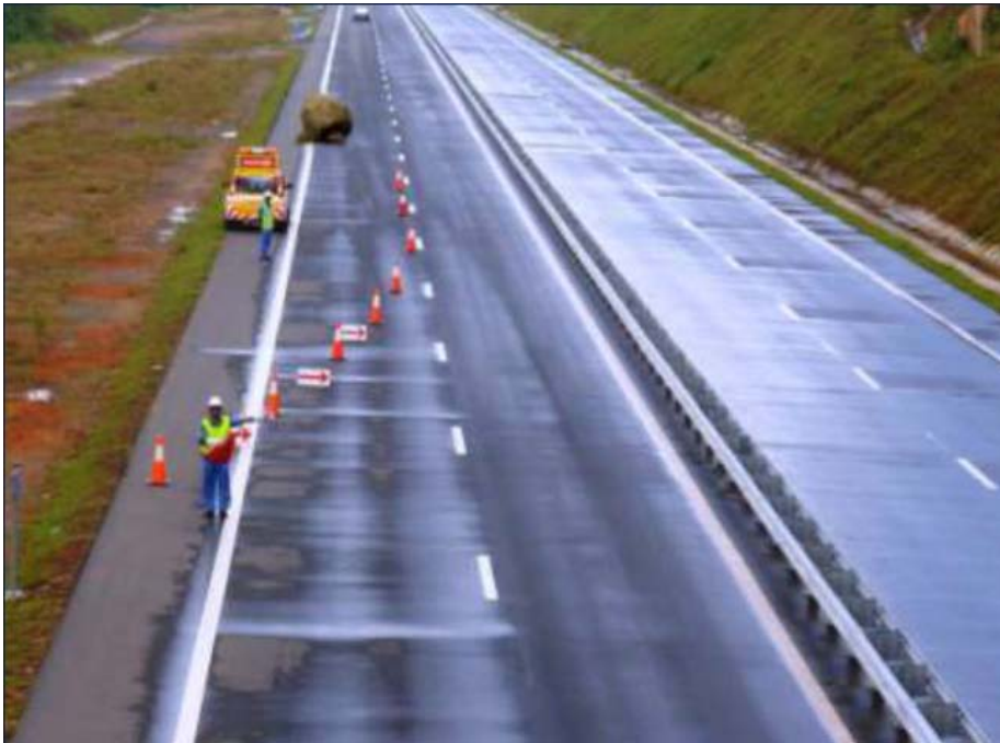
Field training on lane closure in emergency case (Sri Lanka)
