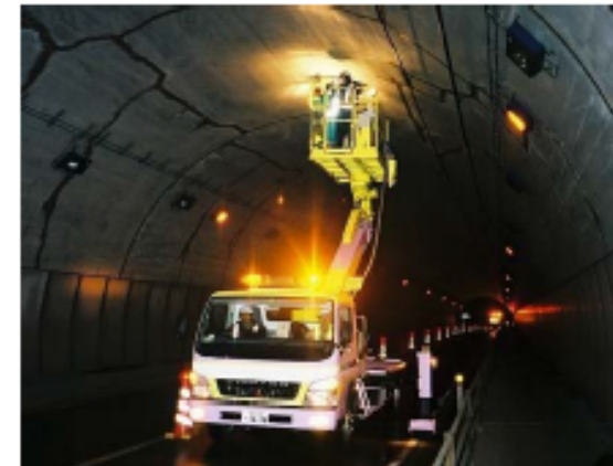
Close-range visual search for cracking
