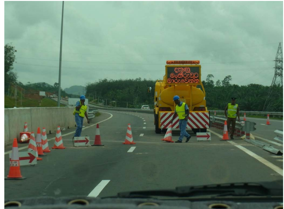
Actual lane closure in emergency case by staff of Road Development Authority, Sri Lanka
