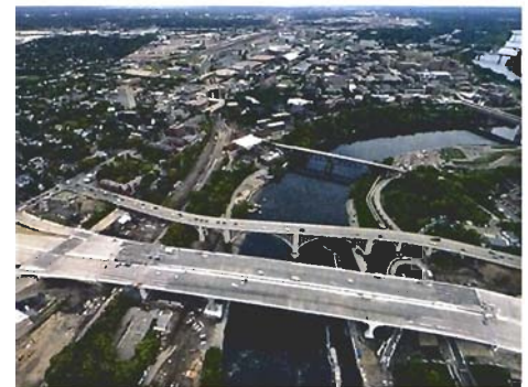
The new I-35W bridge over the Mississippi river in Minneapolis was opened on 18 September 2008.
