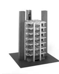
IMAGE THIRTEEN: Louis I. Kahn. American, born Estonia. 1901–1974. Alfred Newton Richards Medical Research Building, University of Pennsylvania, Philadelphia, Pennsylvania. Structure of typical laboratory tower (final version). 1957–65. Model: wood, 28\frac{1}{2} \times 23\frac{15}{16} \times 23\frac{15}{16} " (72.4 x 60.8 x 60.8 cm). The Museum of Modern Art, New York. Gift of the architect
