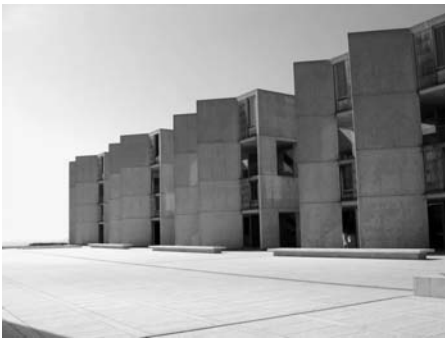
IMAGE TWENTY-SIX: View of study towers, looking west, Salk Institute for Biological Studies, La Jolla, California, 2006. Photograph: Lisa Mazzola
