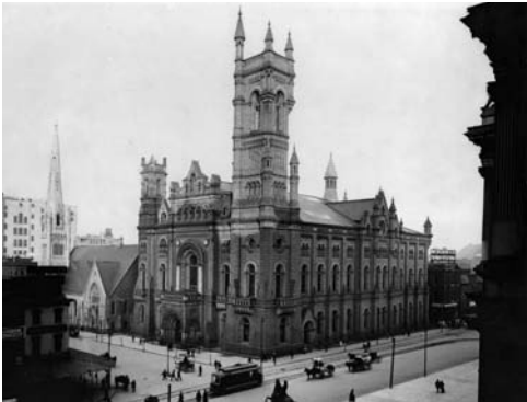
IMAGE ONE: Masonic Temple, Broad and Filbert Streets, northeast corner, Philadelphia, Pennsylvania, c.1902. The Print and Picture Collection, The Free Library of Philadelphia
