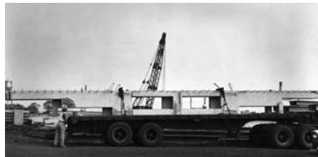
IMAGE FIFTEEN: Pre-cast beam during transport, Alfred Newton Richards Medical Research Laboratories, University of Pennsylvania, Philadelphia, Pennsylvania. The Louis I. Kahn Collection, University of Pennsylvania, and the Pennsylvania Historical and Museum Commission. Photograph: Ronald C. Binks
