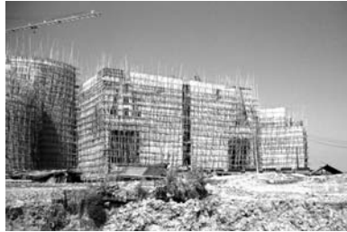
IMAGE THIRTY-THREE: Construction photo, National Assembly Building, Sher-e-Bangla Nagar, Dhaka, Bangladesh, c. 1970. Louis I. Kahn Collection, University of Pennsylvania, and the Pennsylvania Historical and Museum Commission
