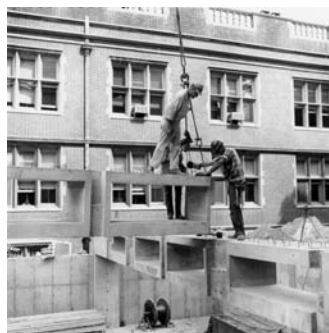
IMAGE SEVENTEEN: Construction photo, Alfred Newton Richards Medical Research Laboratories, University of Pennsylvania, Philadelphia, Pennsylvania. The Architectural Archives, University of Pennsylvania. Photograph: Marshall D. Meyers
