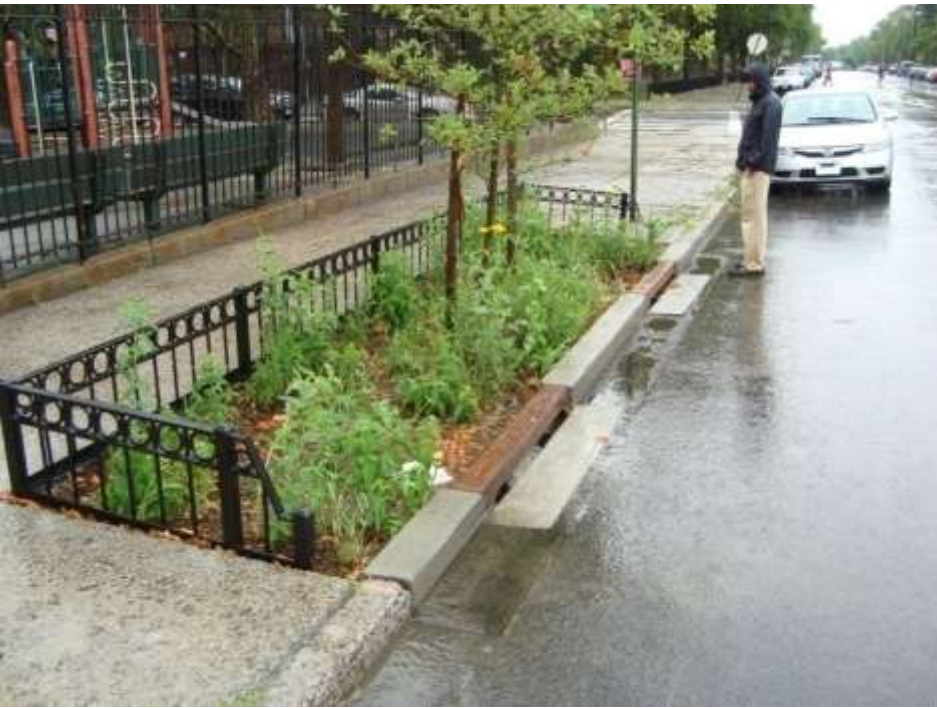
Deep swale with false catch basin at Autumn Ave, Brooklyn
