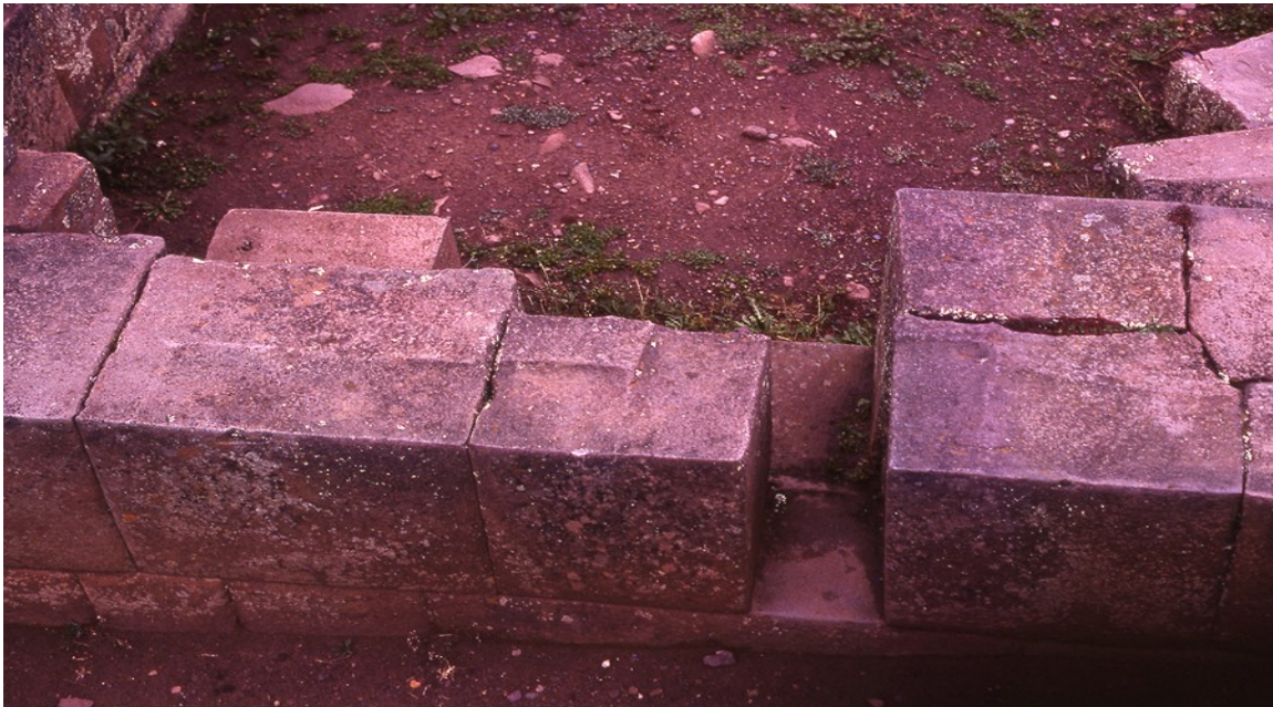
Fig. 5. This dismantled wall from Pisac clearly shows on the upper face of stones the irregular “impressions” of the overlying stone blocks taken away. How were they produced?
