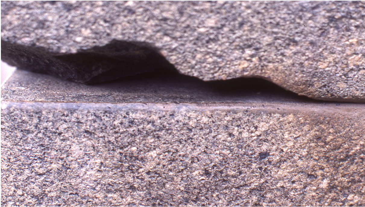
Fig. 8. In this stone junction from Sacsayhuaman (compare fig. 2) part of upper stone is missing and this gives visual access to the surface of the original stone junction, which is much more elaborate and shiny, compared to the rest of the stone surfaces, which were hammered or maybe also polished.
