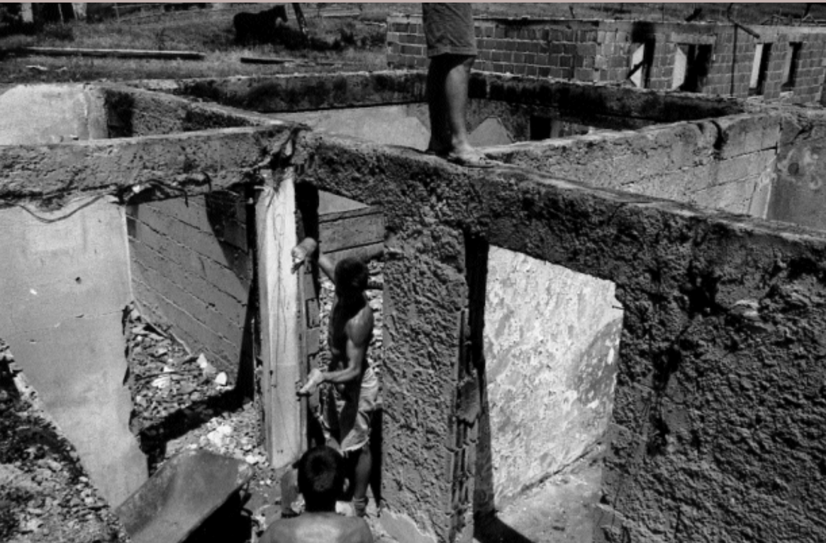
Clearing away the rubble, Studenica, July 1999
