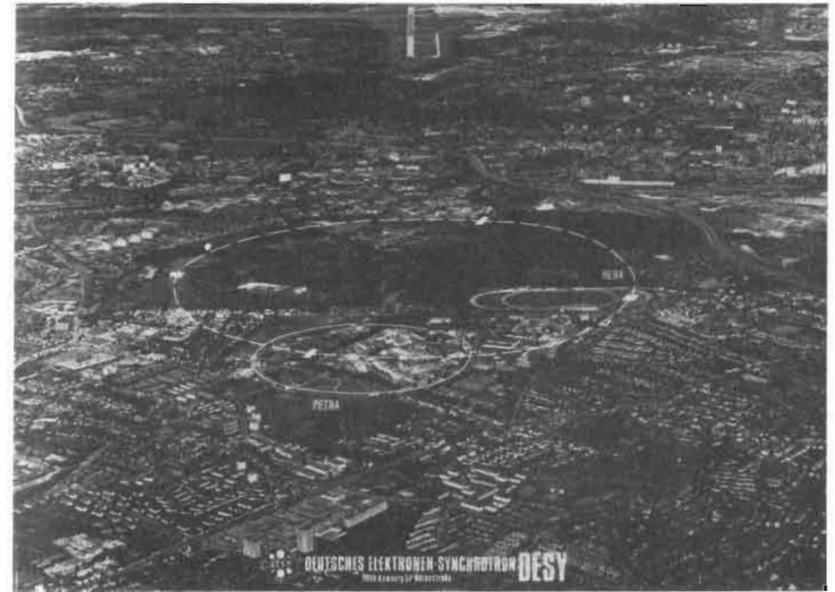
Fig. 6.7: Aerial view of the DESY-accelerator complex in Hamburg where as of 1990 electrons and protons will be made to collide with ultrahigh energy in the accelerator facility HERA presently under construction.
