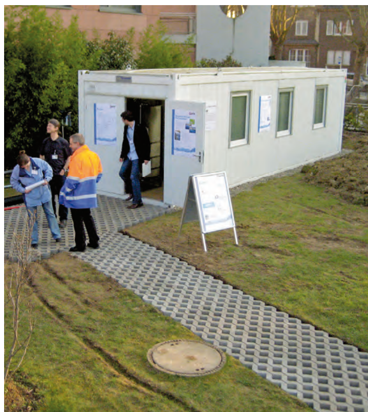
Luxemburg pilot facility
