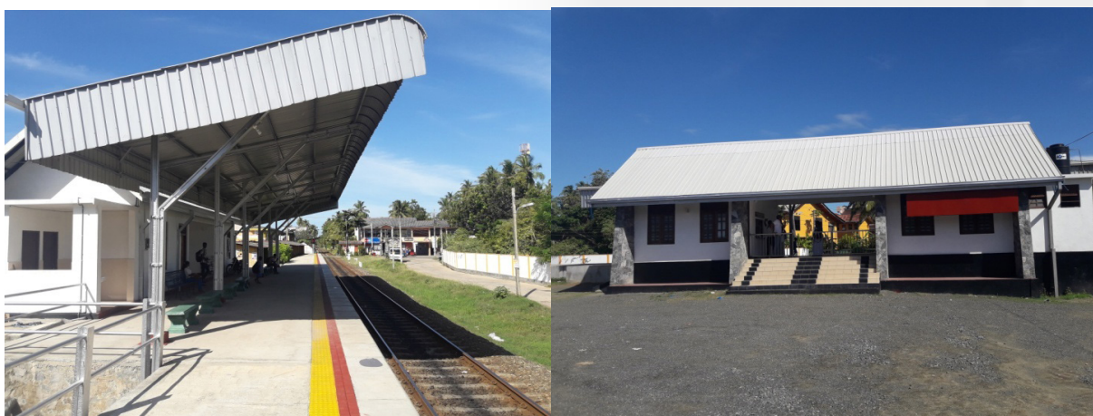
Newly constructed Habaraduwa railway station
