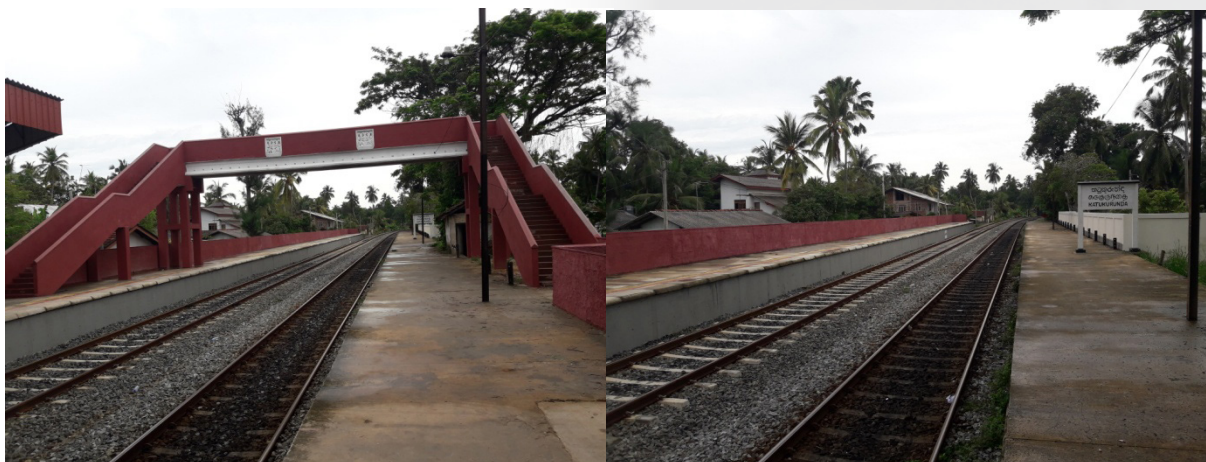
Newly constructed overhead bridge and platform at Katukurunda railway station
