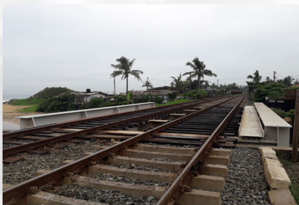
Newly repaired Angulana Bridge
