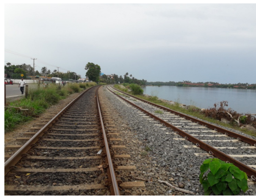
Newly constructed double line between Kaluthara South and Payagala stations
