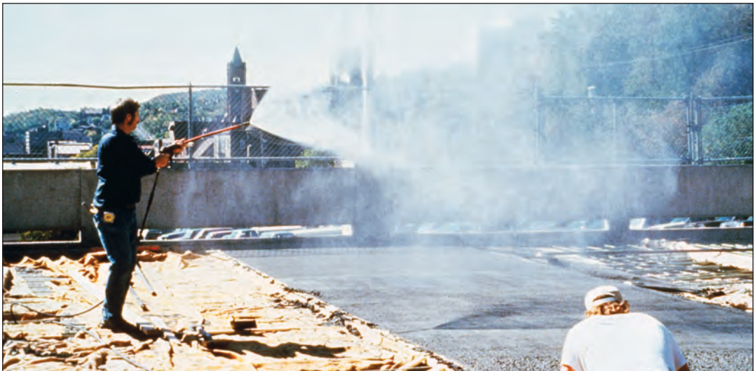
FIGURE 7.5A. Proper fogging of silica-fume concrete in a parking structure to increase humidity and prevent drying of the concrete surface.
