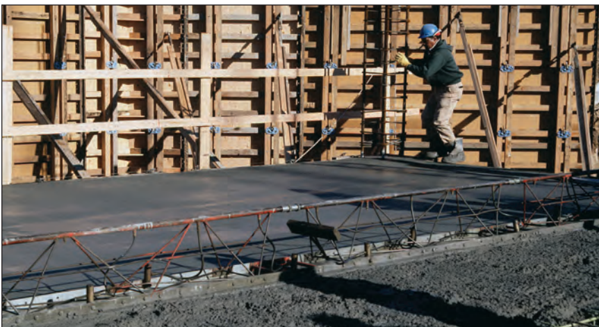
FIGURE 7.15B. Consolidating silica-fume concrete using a vibrating truss screed.
