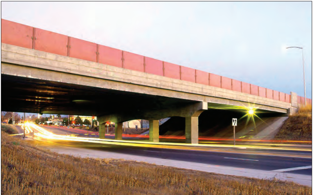
FIGURE 3.9. High-performance concrete bridge. In this bridge in Colorado, high-strength concrete was used to increase span length to eliminate two piers and to increase clearance under the bridge. For more information on this bridge, see the article by Leonard (1999).
