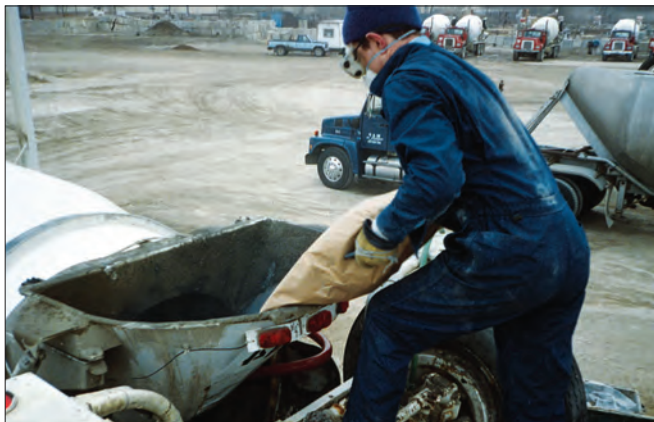
FIGURE 6.8. Emptying a bag of densified silica fume into a truck mixer.
