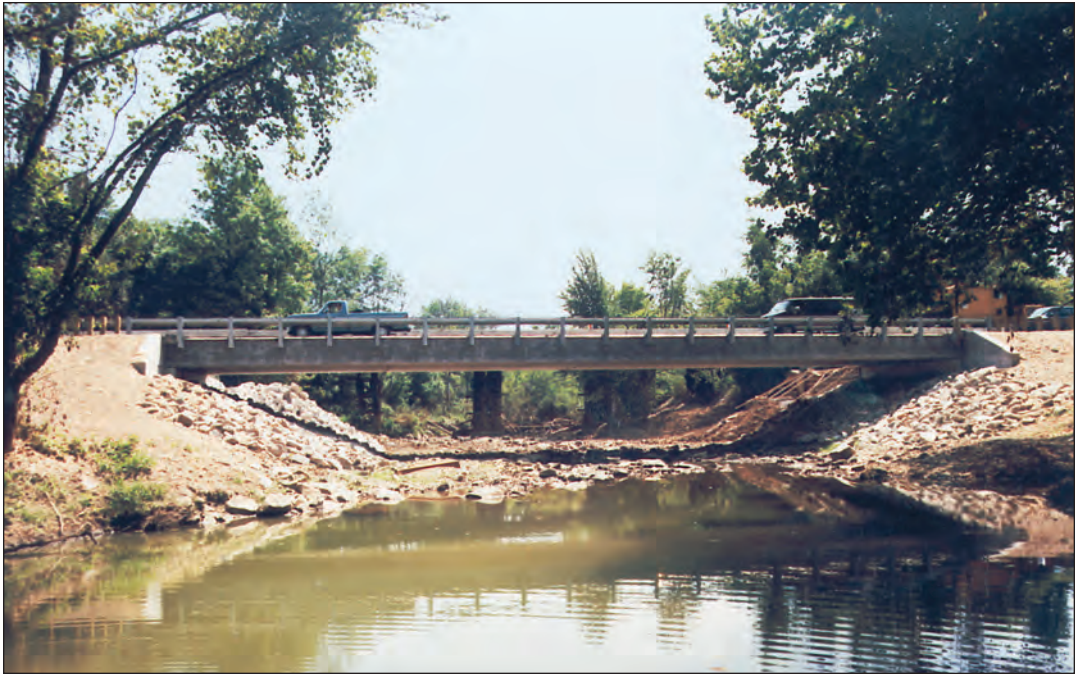
FIGURE 3.7. High-performance concrete bridge. In this bridge in Ohio, high-strength concrete was used to increase span length and eliminate a pier in the river. For more information on this bridge, see the article by Miller (1999).
