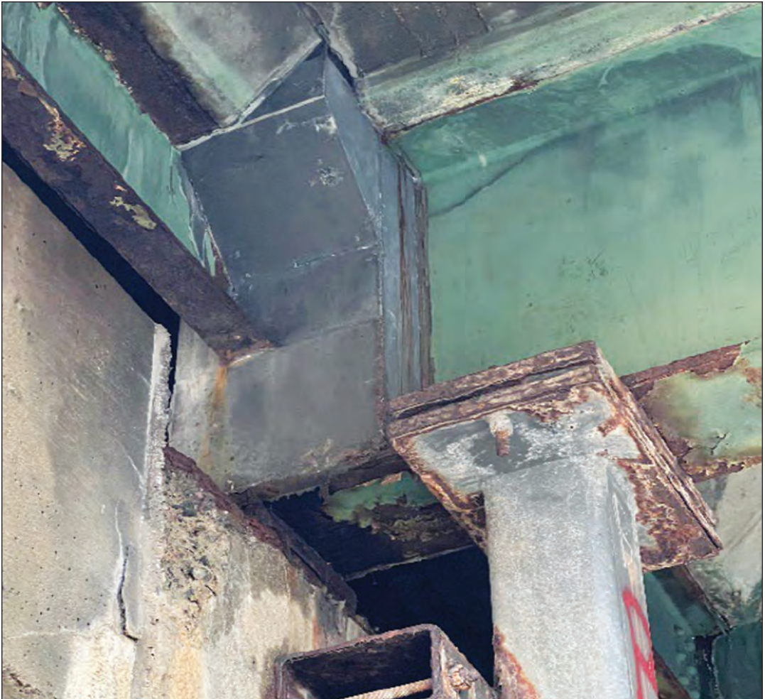
FIGURE 3.22. End of steel bridge beam after repair using UHPC. (FHWA 2022)
