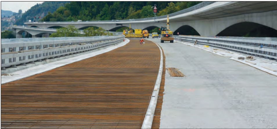
FIGURE 3.24A. Chillon Viaduct deck prepared for overlay with UHPC concrete.
