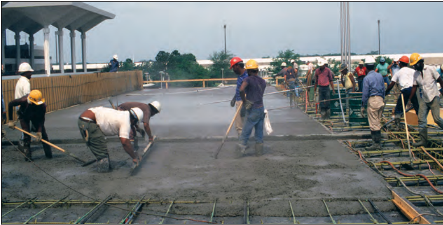
FIGURE 7.15A. Consolidating silica-fume concrete using a hand screed.
