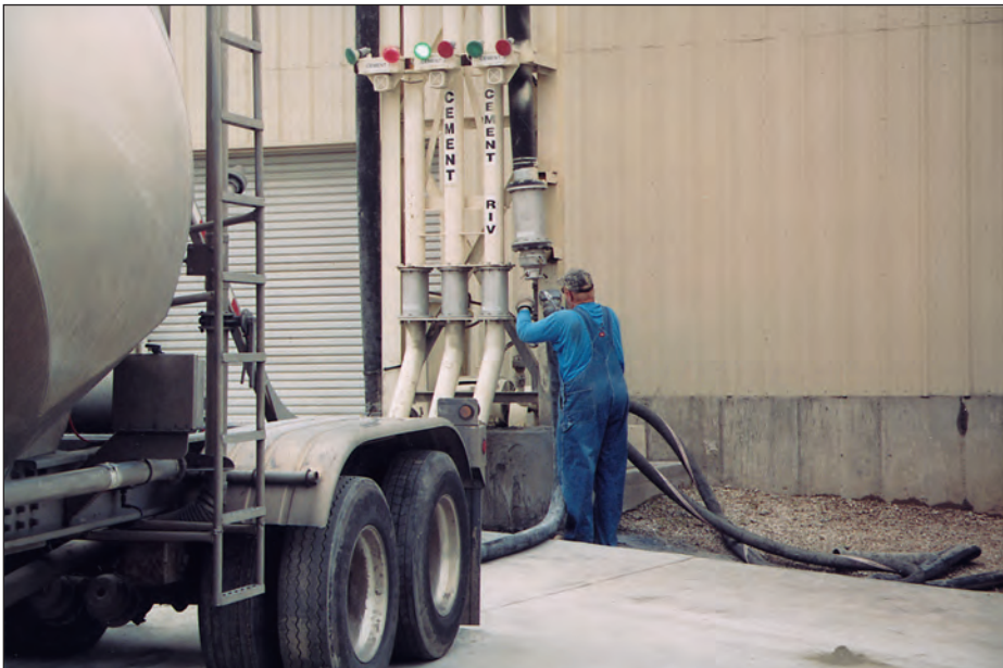
FIGURE 6.5B. Connecting rubber hose from tanker to rubber fill hose of silo.
