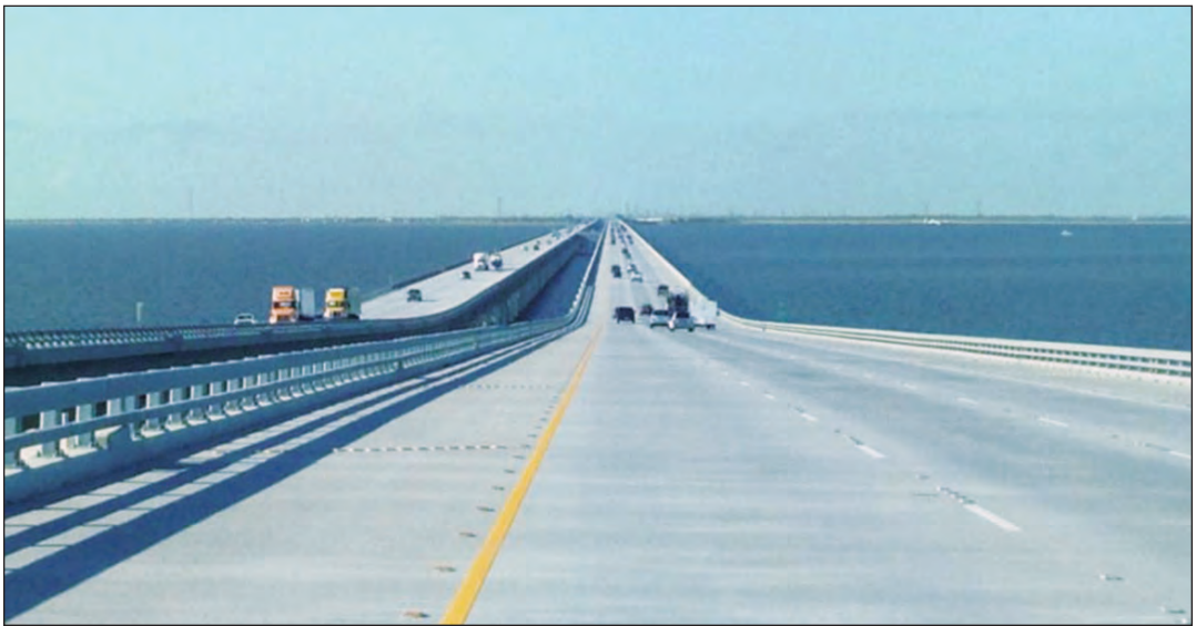
FIGURE 3.15. After Hurricane Katrina damaged the I-10 Highway into New Orleans, the Louisiana Department of Transportation designed its replacement for longer service life with increased concrete durability, specifying a very low rapid chloride permeability rating on its new concrete structure.
