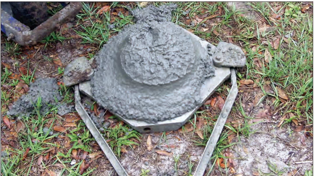
FIGURE 5.2. Slump of concrete placed on the tank dome was approximately 200 mm.
