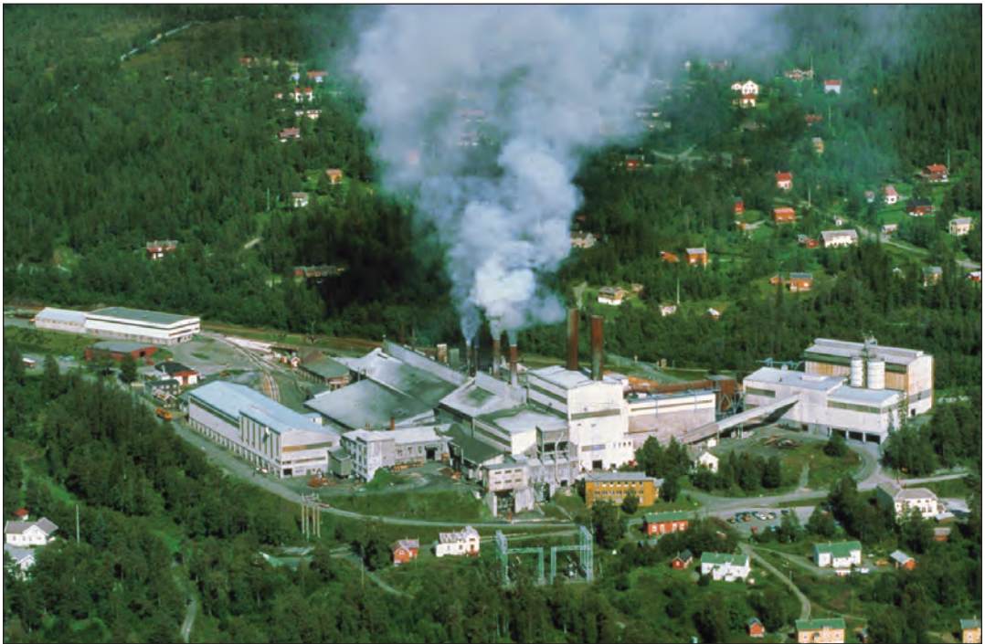
FIGURE 1.2. Smelter before installation of equipment to collect silica fume. The “smoke” is silica fume being released to the atmosphere.
