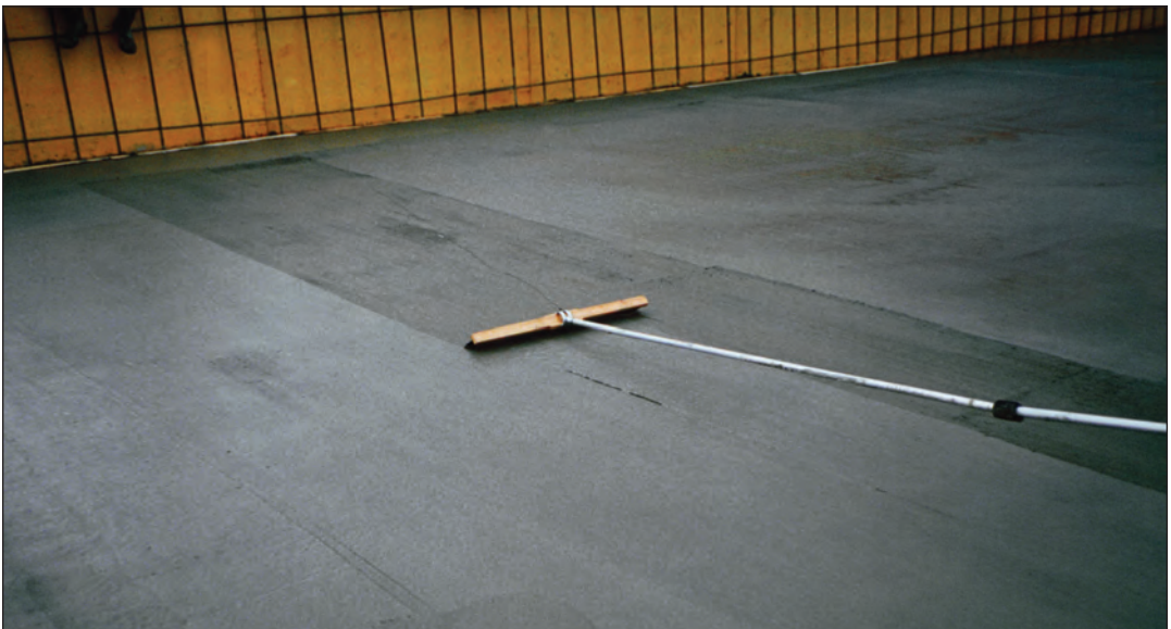
FIGURE 7.17C. Brooming of a silica-fume concrete surface. In this case, the broom has a wire attached to it to lift it off the surface for travel from right to left in the photo. The texture is applied by pulling the broom from left to right.
