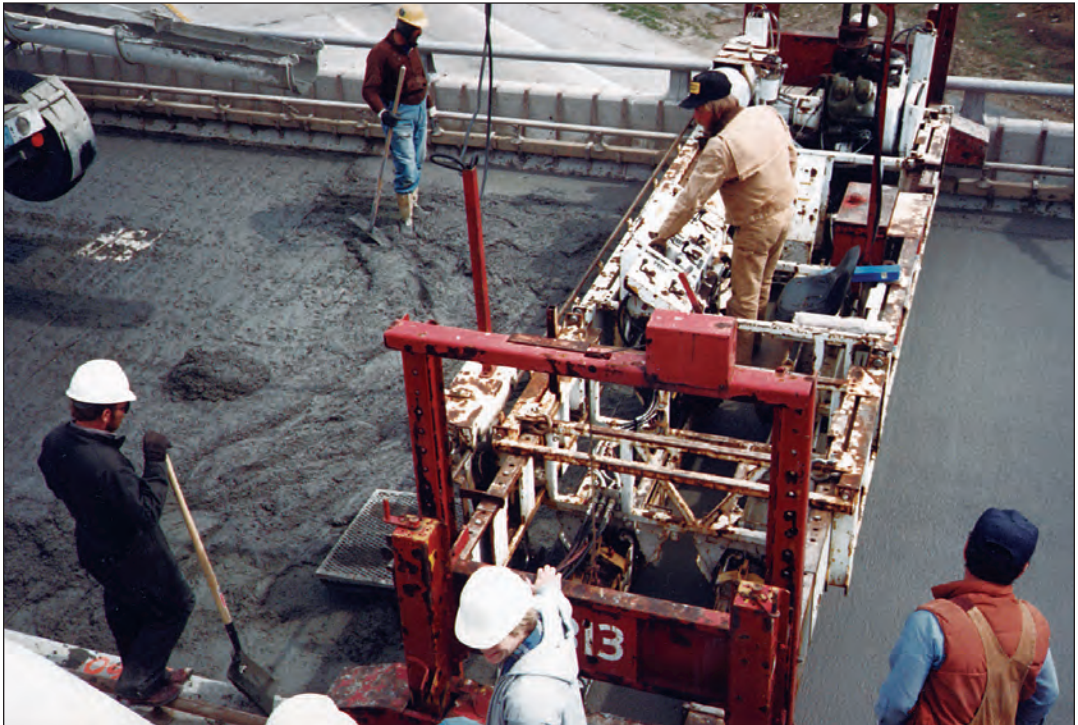
FIGURE 7.9. Bridge deck machine being used to place silica-fume concrete overlay.
