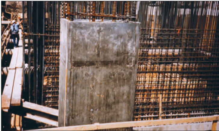
FIGURE 3.6. High-strength silica-fume concrete column in a high-rise structure.
