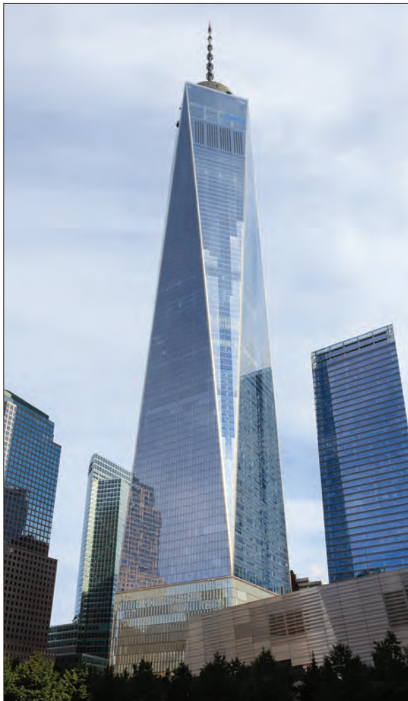
FIGURE 3.19. For the World Trade Center, high strength was initially the foremost goal for hardened concrete properties. The ability to achieve long-distance, vertical, single-stage pumpability of SCC coupled with consolidation around congested reinforcement was ultimately a more important goal in the fresh state of this concrete. This concrete mixture also was noted for its low-carbon footprint.
