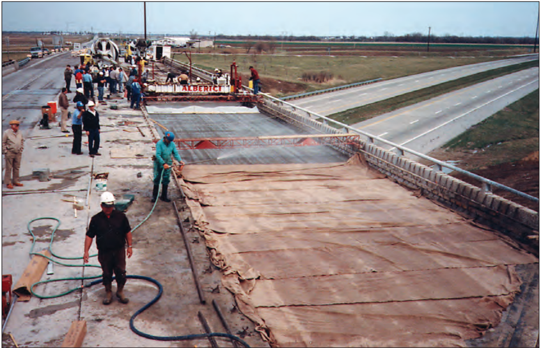
FIGURE A.1. Bridge deck project. Mixture proportions for a concrete that could be used on this project are developed in Example 1.
