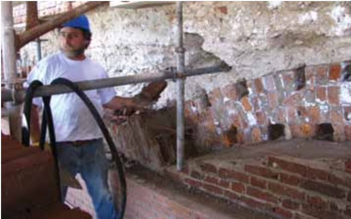
Figure 9: Tie bricks let into the undamaged vaulting tie the new vaulting into the old. The coral concrete is seen above.
