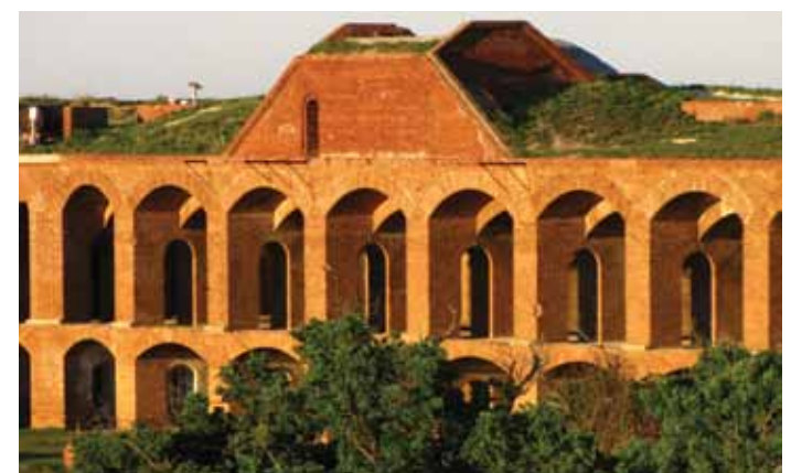
Figure 3: Arches and vaults composed of 16 million bricks surround inner cores of coral concrete.
