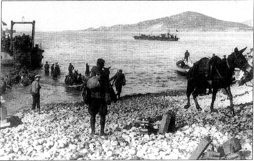
Unloading mules and supplies during the Alhucemas landing.
