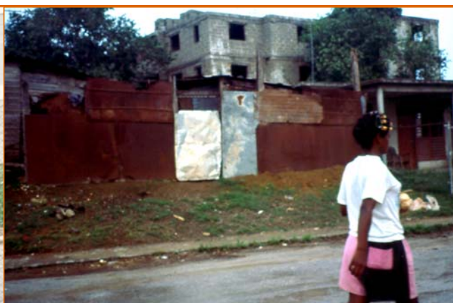
Photo 20. Before and After in La Güinera: Shantytown Housing with New Buildings Behind
