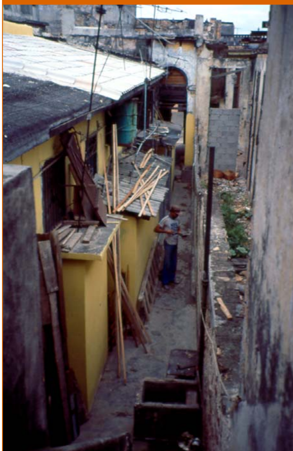
Photo 3. Atarés Tenements where Residents have Expanded their Units into the Narrow Courtyard. The Leaking Roof is being Repaired with Roof Tiles Produced on Site with Low-cost Technology
