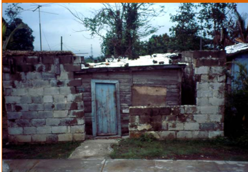
Photo 7: A Shantytown Unit in the Process of Replacement by a Solid, Masonry Dwelling
