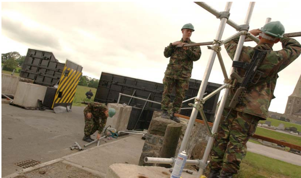
Figure 7-3: Construction of the Roadblock at Drumcree for the 2003 Marching Season
