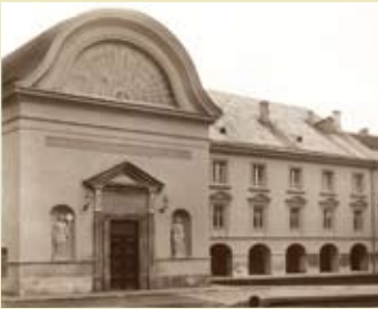
▲ The Aula (or Hall) of the University of Vilnius in the Grand Courtyard in 1929. After the reestablishment of the University, in August 1919 Józef Piłsudski confirmed the restitution of old University buildings on Universiteto, Skapo, Pilies and Šv. Jono streets to Stephanus Bathoreus University, as well as the buildings on Šv. Onos, Bokšto, Savičiaus streets and Šv. Kazimiero alley previously belonging to the Bernardinian and Augustinian monasteries, the building of the former Collegium nobilium on Pilies street, the building of the School of Chemistry and Technology on Naugarduko street, the buildings of the Russian Aleksey's Military School of Artillery on Zakreto (later M. K. Čiurlionio) street, the barracks on Šv. Ignoto street, Frank's house on Didžioji Street and other smaller buildings in the Old Town. Those buildings were used for auditoriums and study rooms, library, offices for the administration and flats for professors and other university staff.
