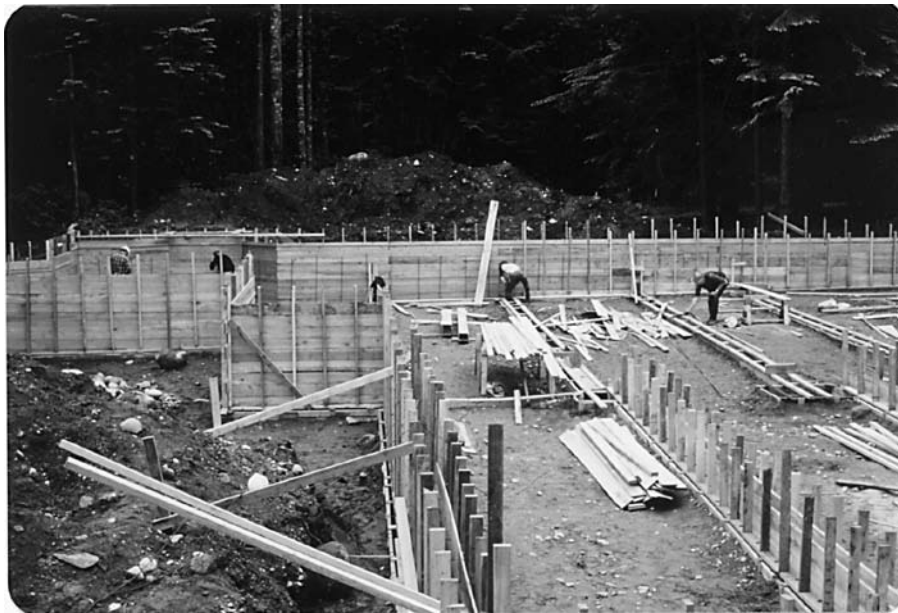
Forming the concrete walls.
