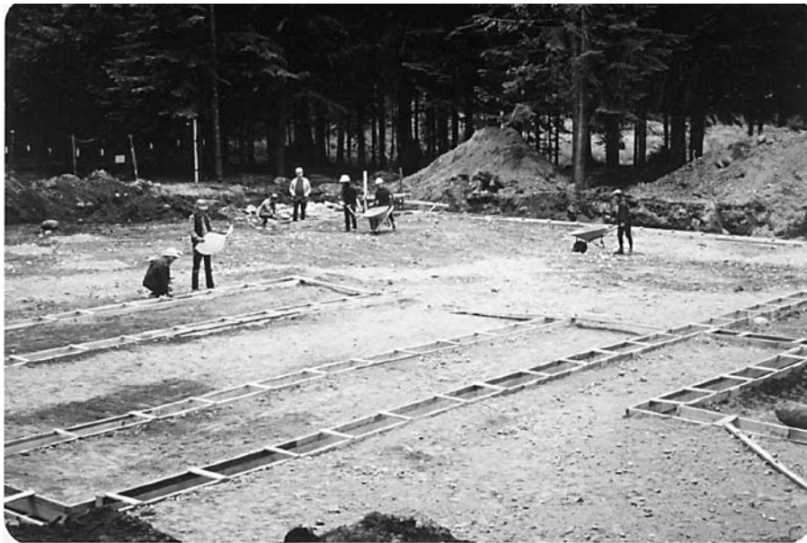
Laying the footing of the main hall.
