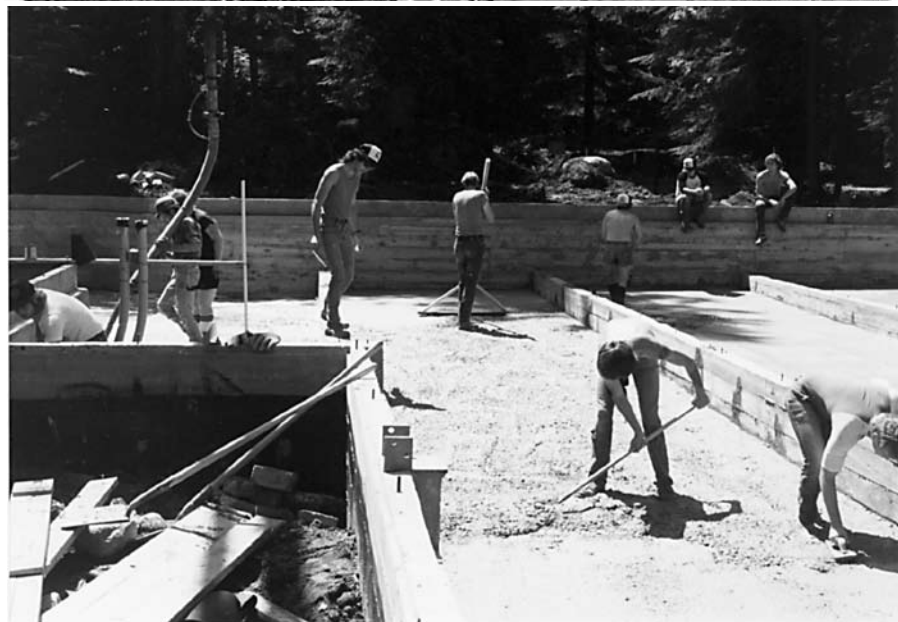
Leveling the skin coat in the crawlspace area.
