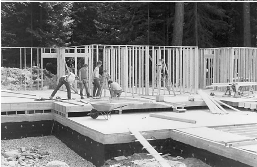
Framing the walls. Notice gravel for drain tiles.
