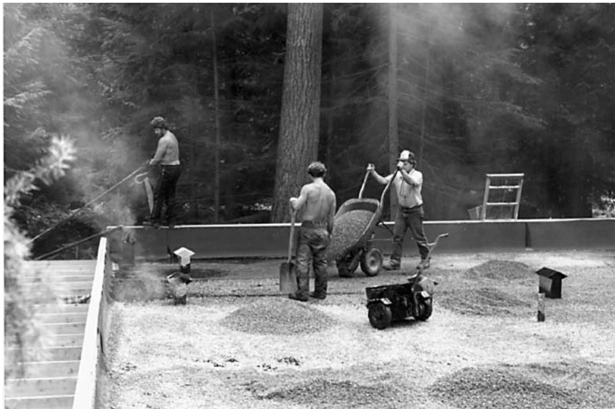
Whonnock Roofing crew puts tar and gravel on the flat roof.
