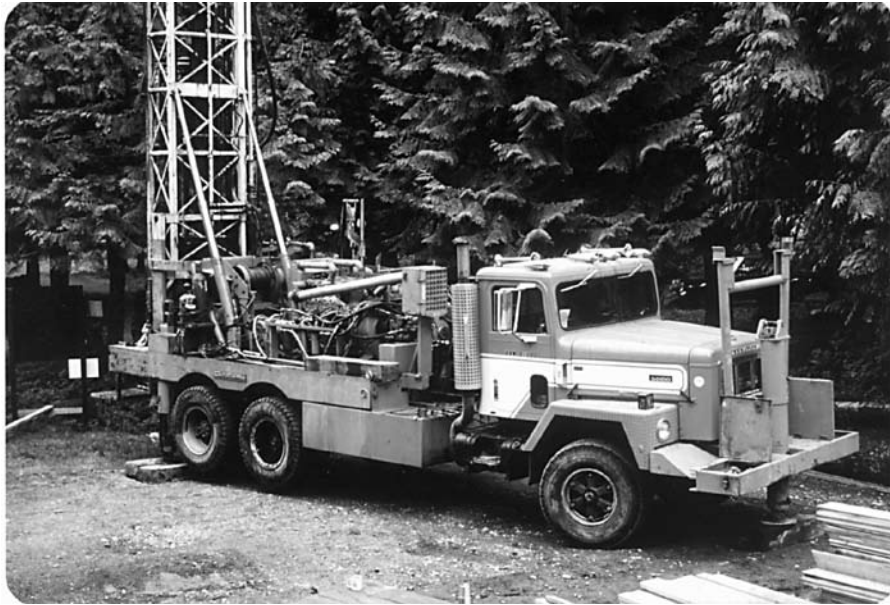
Drilling the well for the centre.
