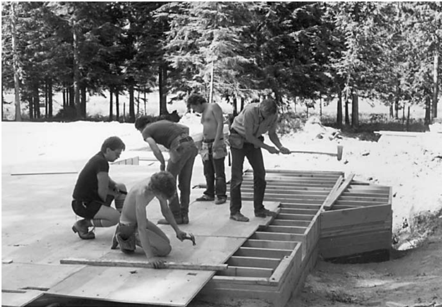
Putting down the sub-floor on the pre-school area.
