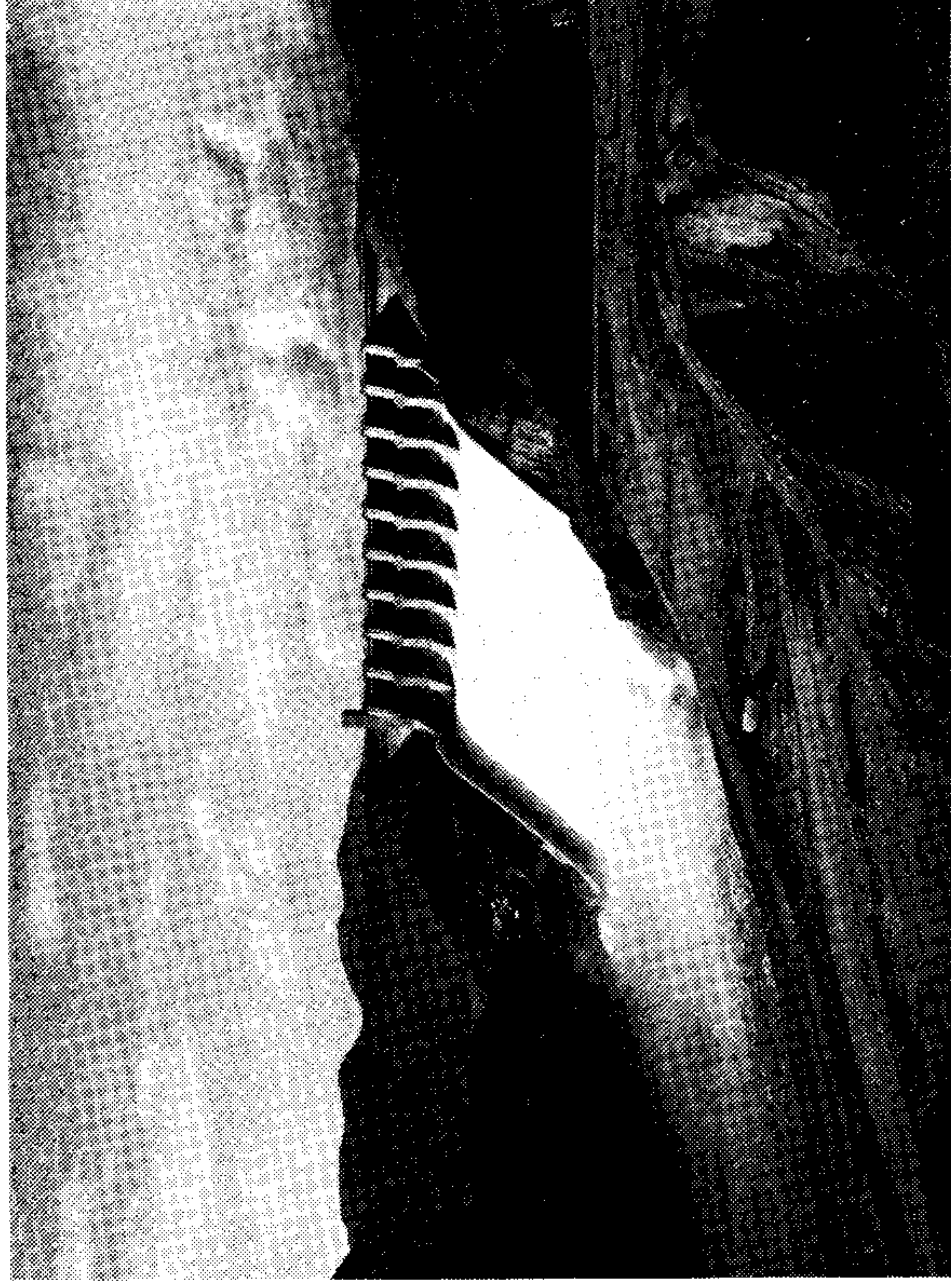
In the 20th and 21st centuries, water-management systems requiring significant energy inputs are a prerequisite for sufficient improvement of land. Above: the Tarbela dam system in Pakistan.
