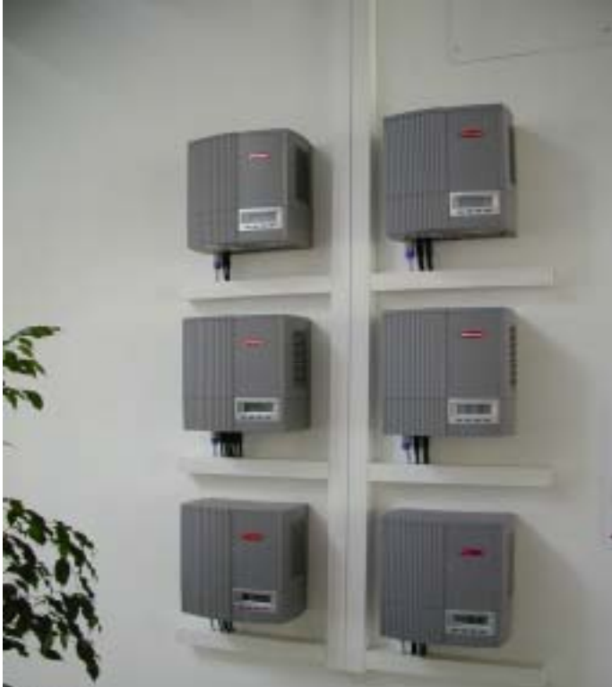
Figure 17. Simplified European Inverter Installation.
