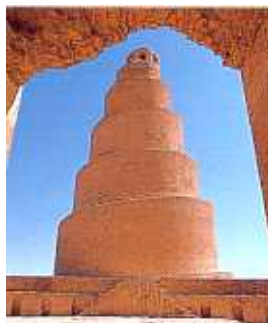
2. The Malwiya minaret , Samarra, Iraq, mid-ninth century. This 50-meter (160') helicoidal tower of sun-dried and baked brick may have been modeled on ancient ziggurats. It symbolizes the power of Islam at the zenith of the Baghdad-based Abbasid caliphate.
