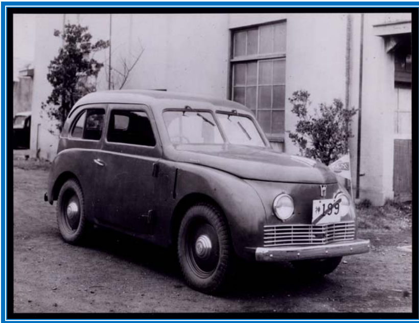
Datsun's first postwar automobile, the DB, appeared in 1949 with essentially a prewar Datsun rolling chassis. The 1950 version was given a larger engine in an effort to advance the design. Overall, however, it was efforts such as this that convinced MITI of the need to learn from tie-ups with competent foreign manufacturers. Original photograph and hood emblem from author's collection.
