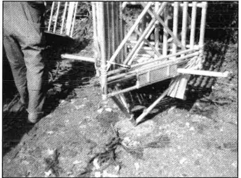
Surveying towers reached their peak in the early 1970s with easy-to-install, prefabricated units. They were later made obsolete by GPS.
