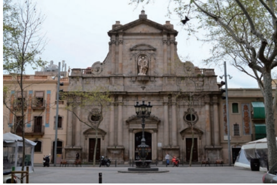
Fig.6 San Miguel del Puerto, a church designed by military engineer Pedro Martín Zermeno in Barceloneta
