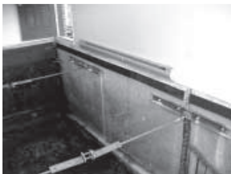
Straightening the foundation wall with tie rods
