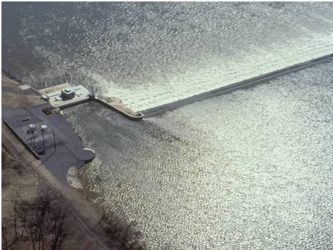
Figure 29. Aerial view of Allegheny Dam 5 and hydropower plant (Photo courtesy of the U.S. Army Corps of Engineers, Pittsburgh).
