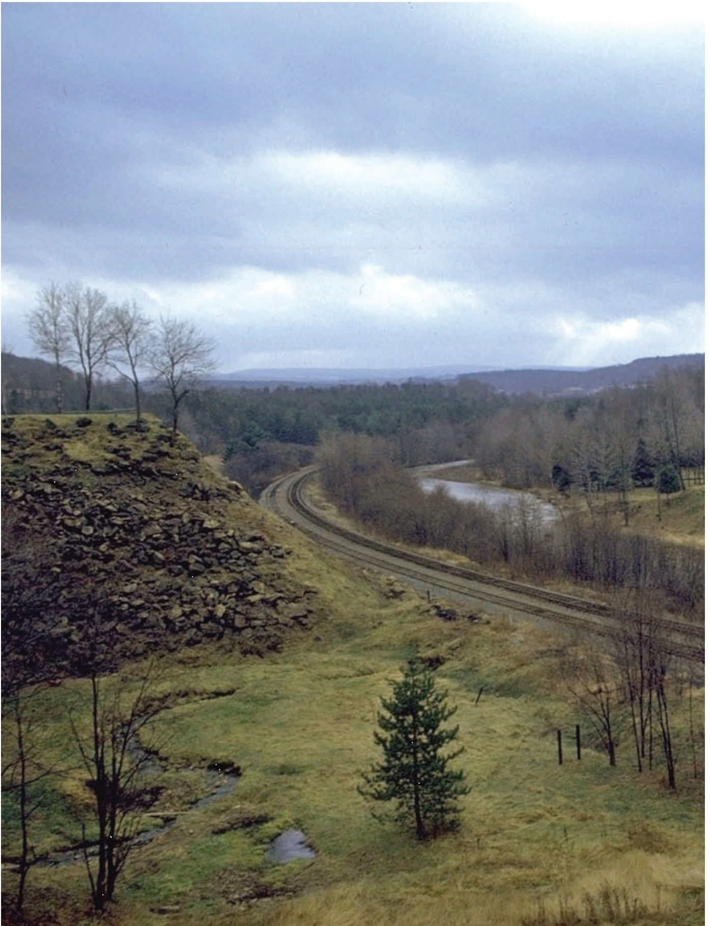
Figure 38. Current photograph of South Fork Dam depicting abutment remnants (National Park Service, 2008).
