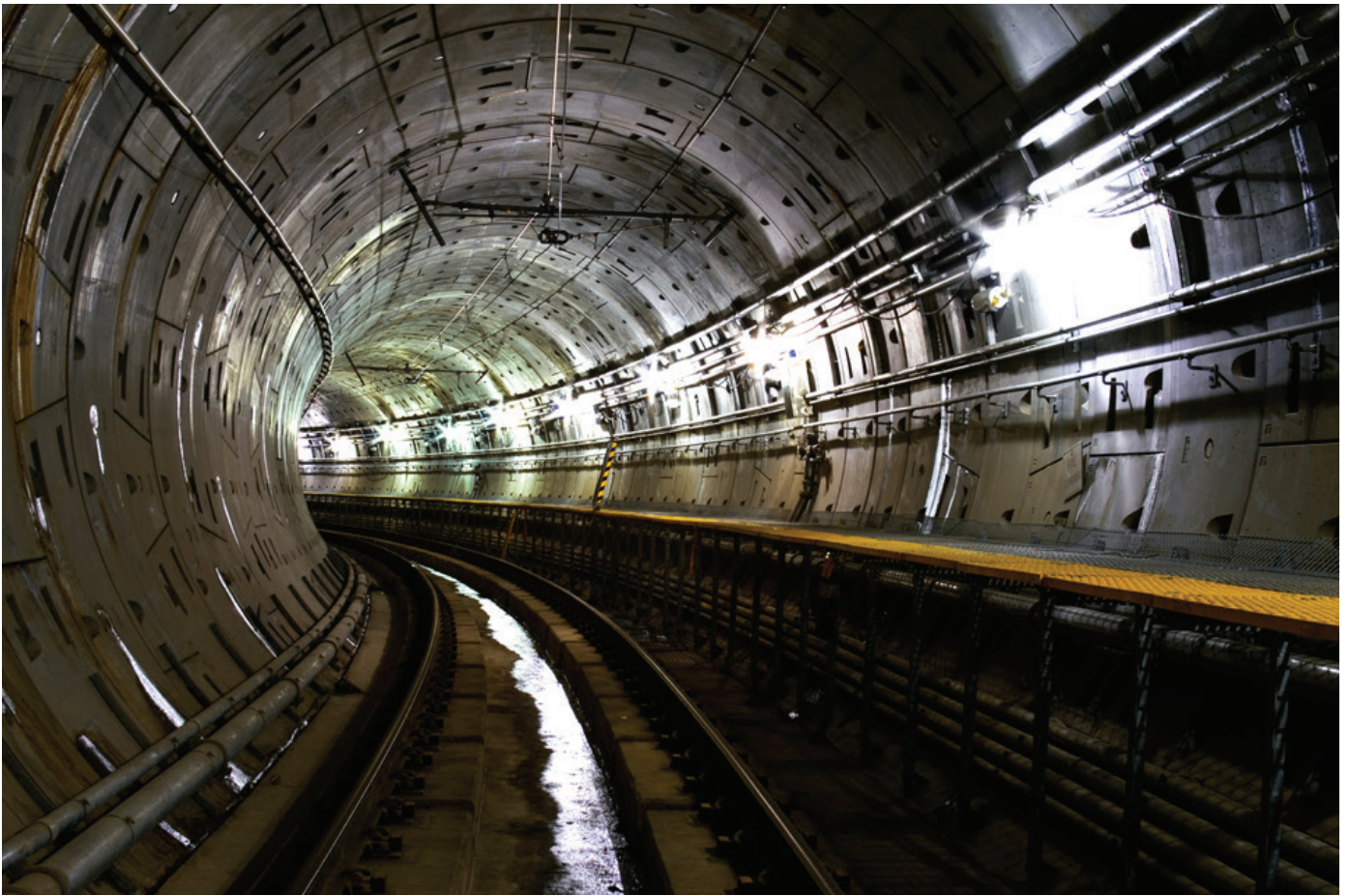
Figure 57. Interior of the completed North Shore Connector Tunnel.
