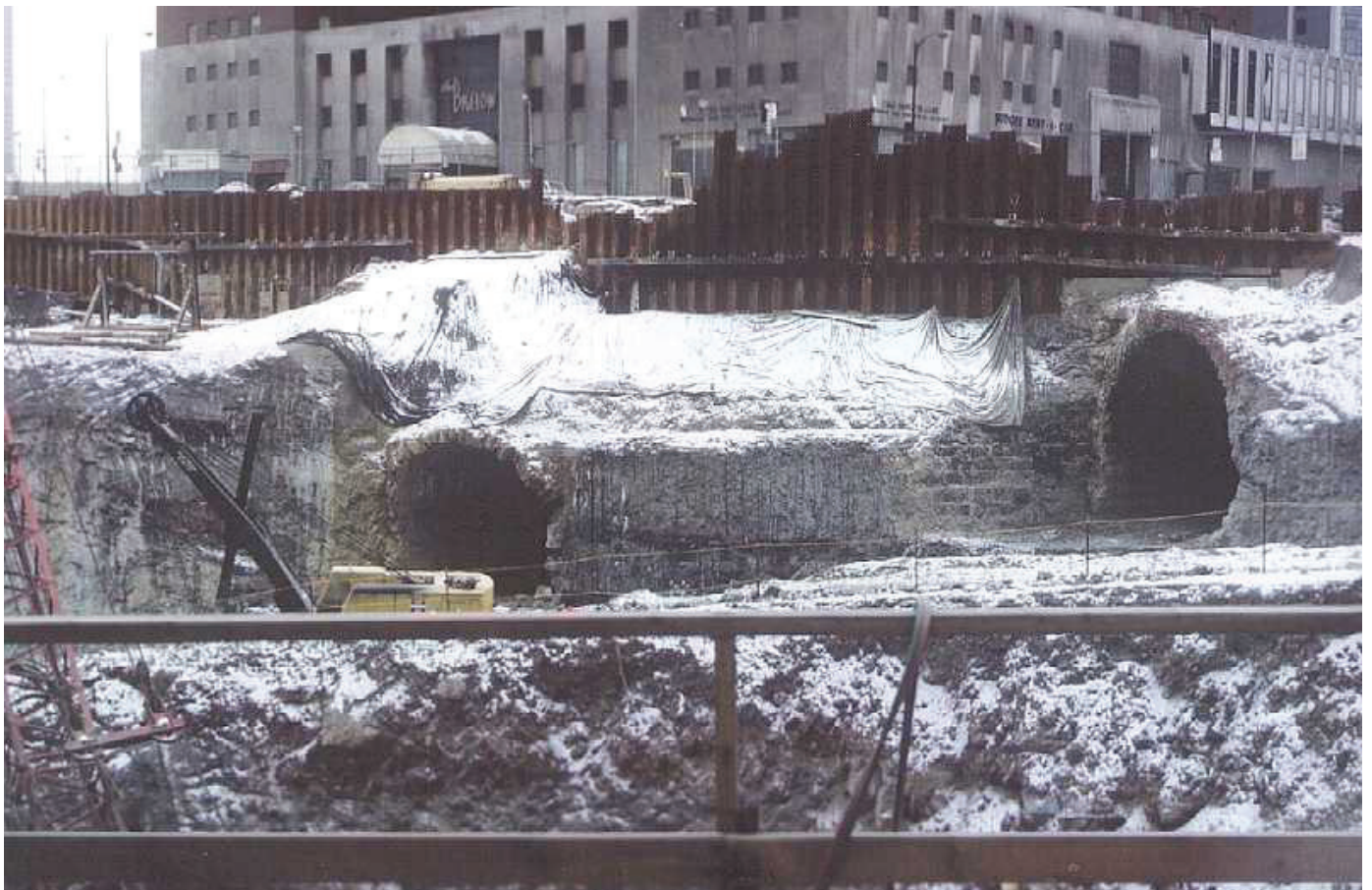
Figure 45. Tunnels exposed during USX Tower foundation construction (Rathke, 1968).
