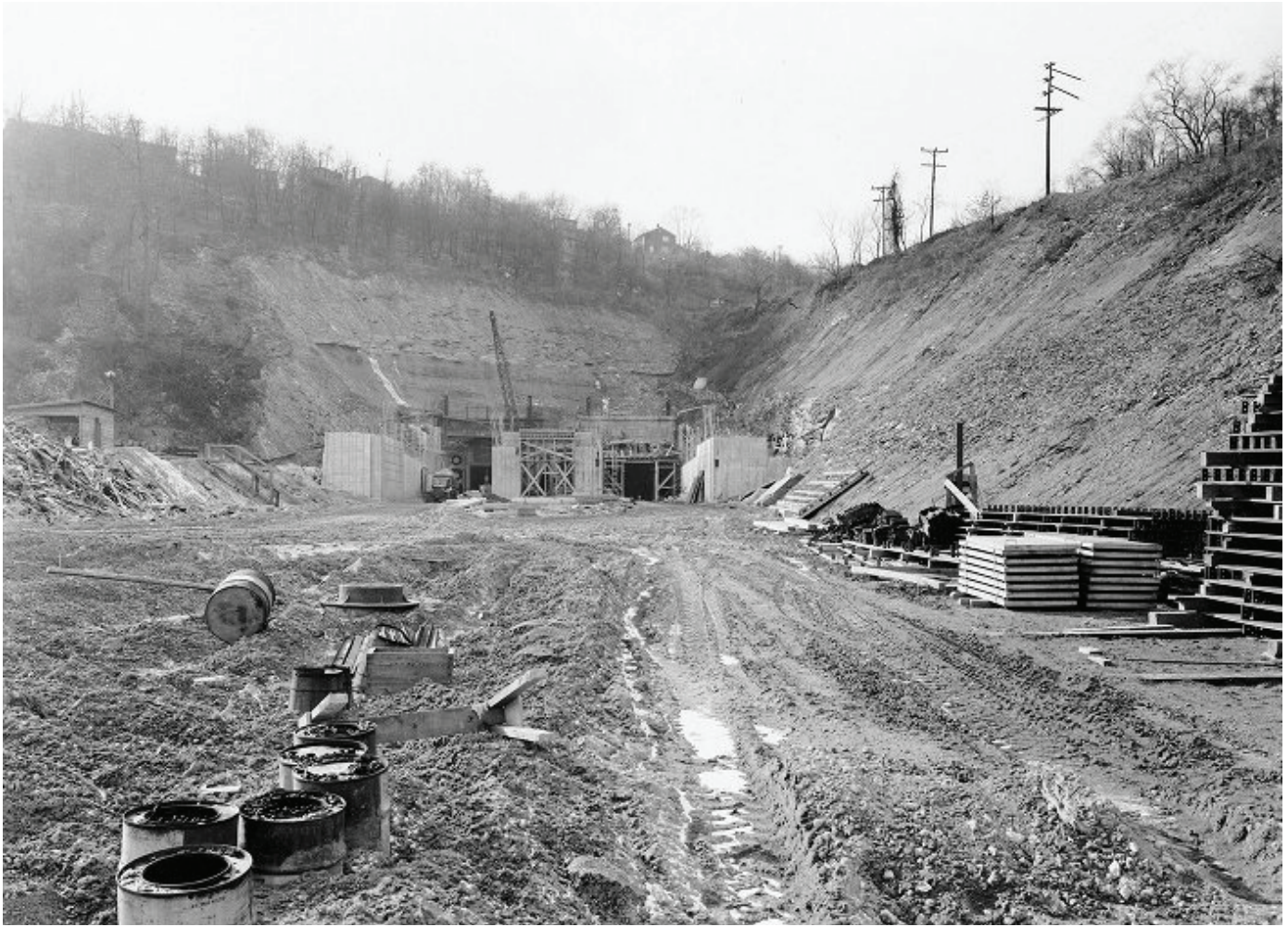
Figure 54. Squirrel Hill Tunnel Construction, 1953 (Collier, 2014).
