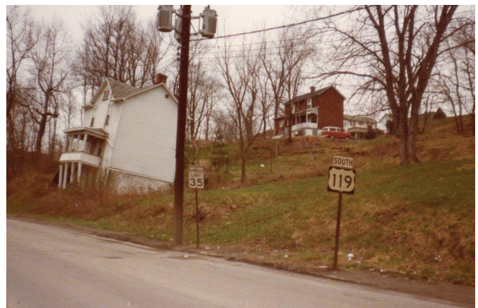
Figure 43. House Damaged by Sinkhole Subsidence – Connellsville, PA (Photo by R. Turka, 1979).
