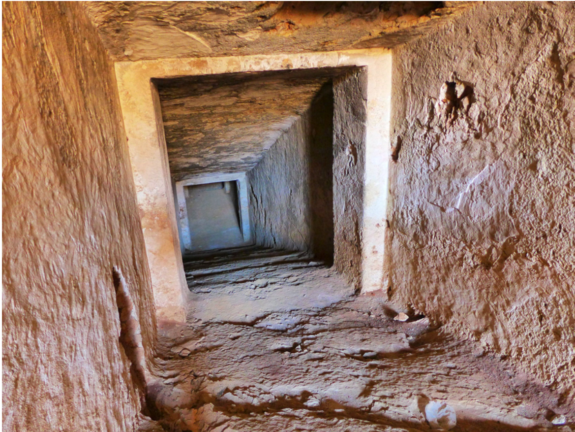
Figure 7. The descent into tomb 29. Large areas of gypsum plaster remain on the walls and ceiling. Photo B. Kemp, 2015.
